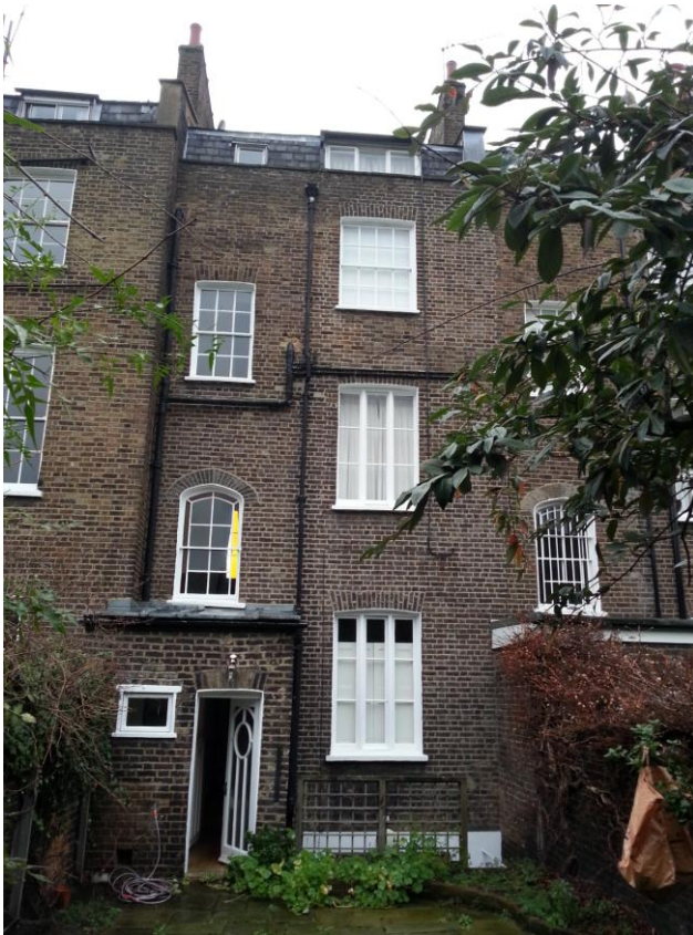
Photo 2: Rear elevation of No. 29 Lonsdale Square
