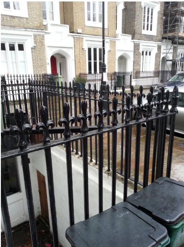
Photo 3: Front railings at No. 29 Lonsdale Square
