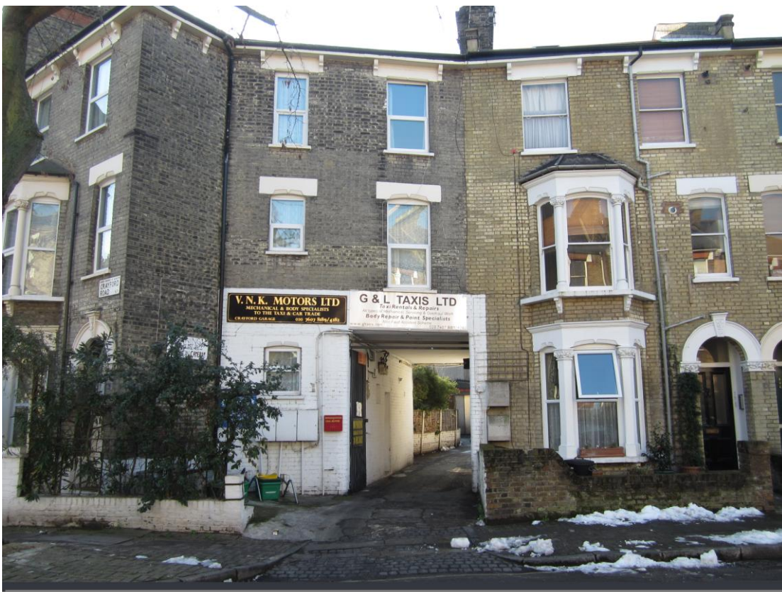
Entrance to site from Crayford Road
