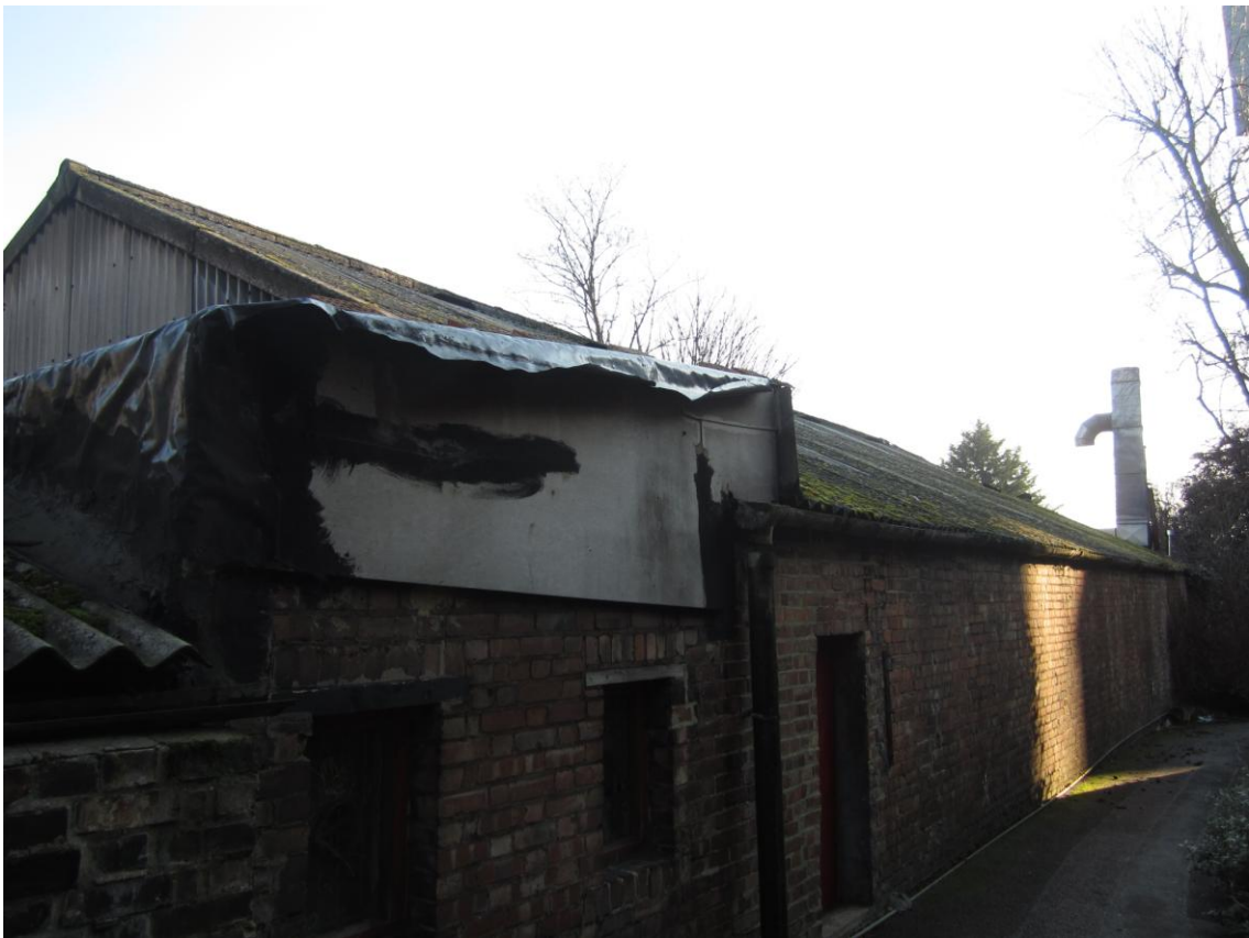
Front and southwest side elevation of garage workshop building
