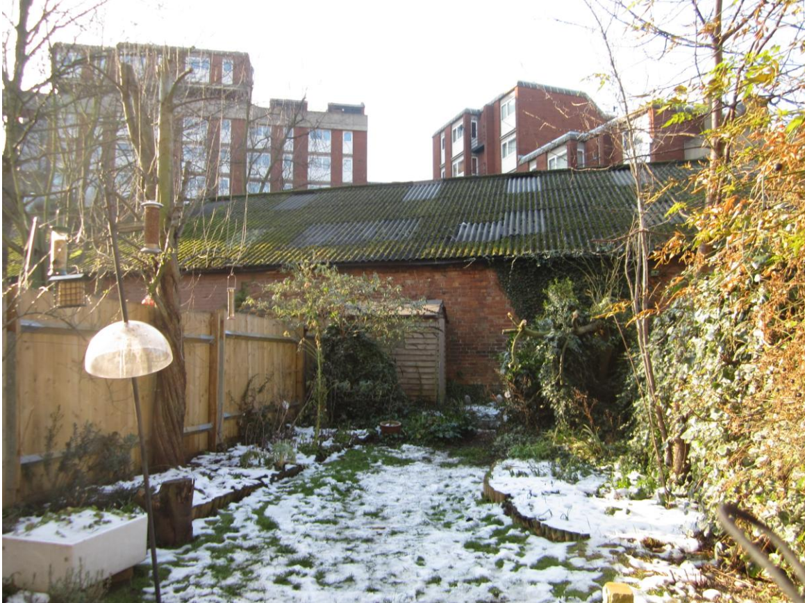
Northeast side elevation of garage workshop building
