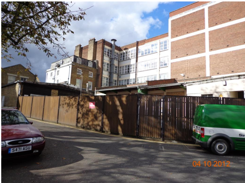
Looking north-west from within the application site capturing the rear elevation of Ladbroke House (LMU), No 60 Highbury Grove and the buildings (and extension) to the rear of No 58 Highbury Grove to be demolished
