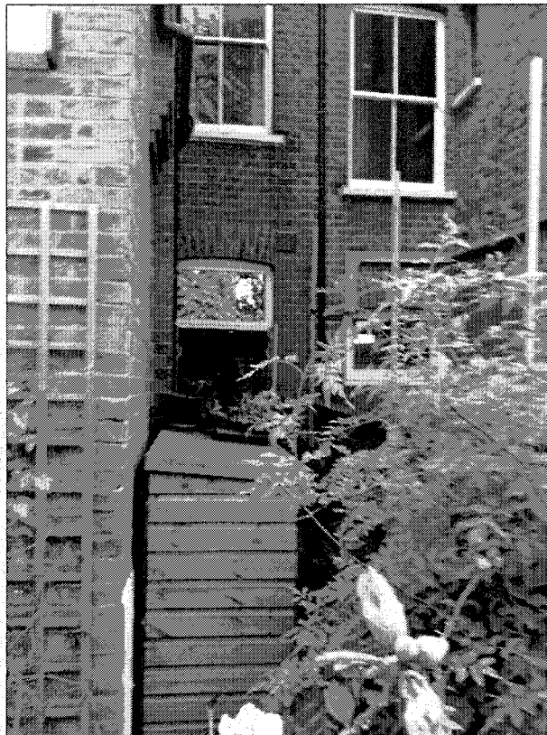
PHOTO 1: VIEW OF REAR ELEVATIONS OF 7 & 9 SOTHEBY ROAD.
