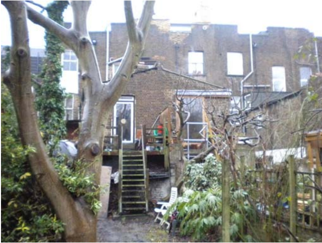
ABOVE: Rear of site
