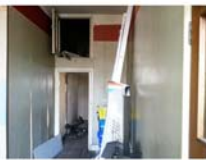
level 2 access to rear extension
