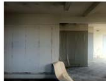
level 3 rear walls
