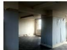
level 3 front east
