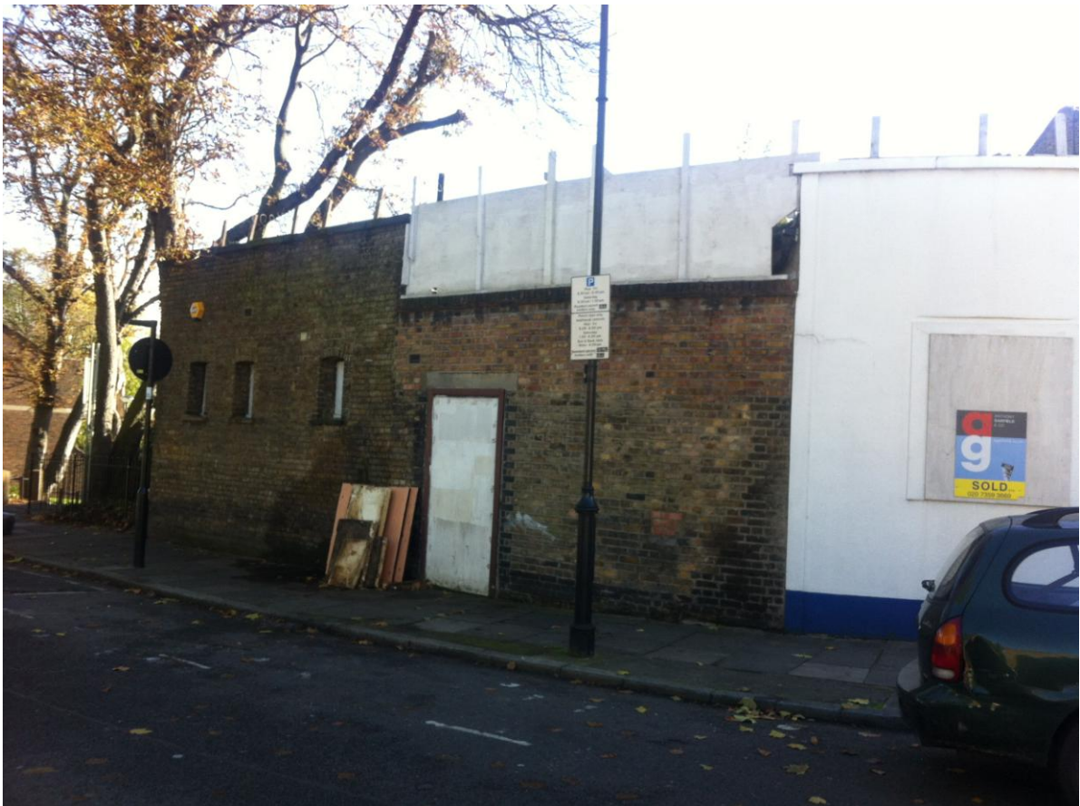
Non-original brick addition to be removed to create courtyard.
