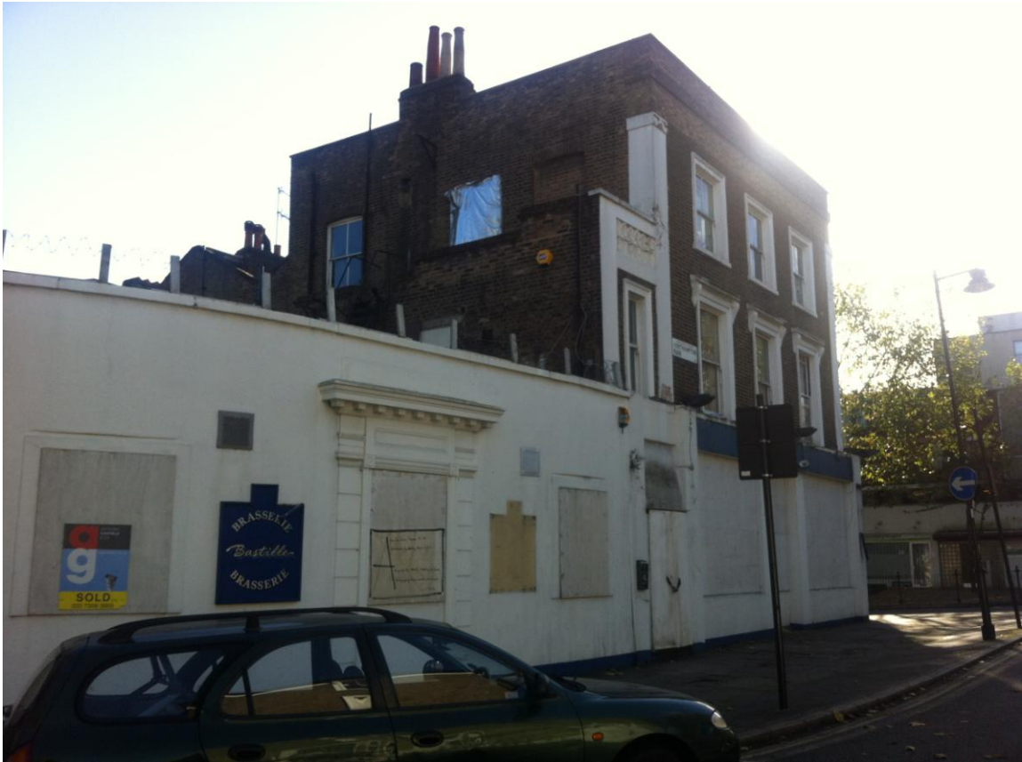
Rear stucco single storey addition to be retained.
