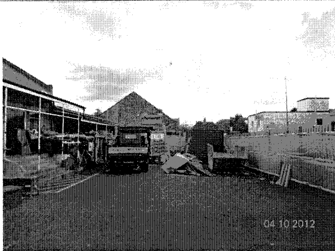
EXISTING YARD TO REAR OF THE COACH HOUSE. BUILDINGS TO BE DEMOLISHED ARE SITED TO THE LEFT.
