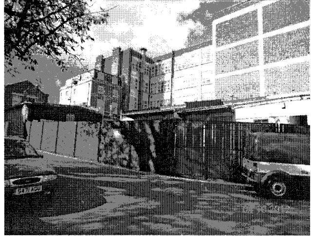
EXISTING EDGE TREATMENT OF SITE ALONG MELODY LANE WITH LADBROKE HOUSE AND 60 HIGHBURY GROVE IN BACKGROUND.
