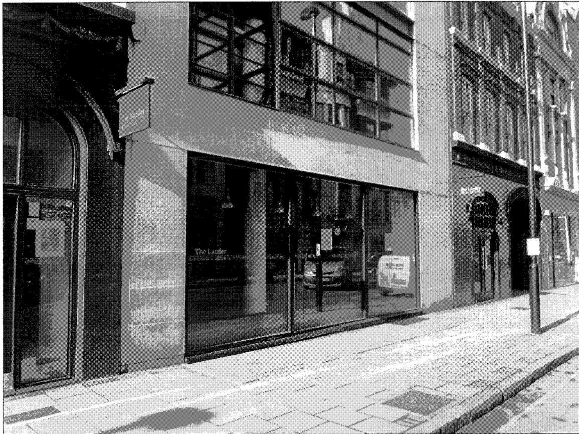
Front elevation of application site viewed looking northwest.
