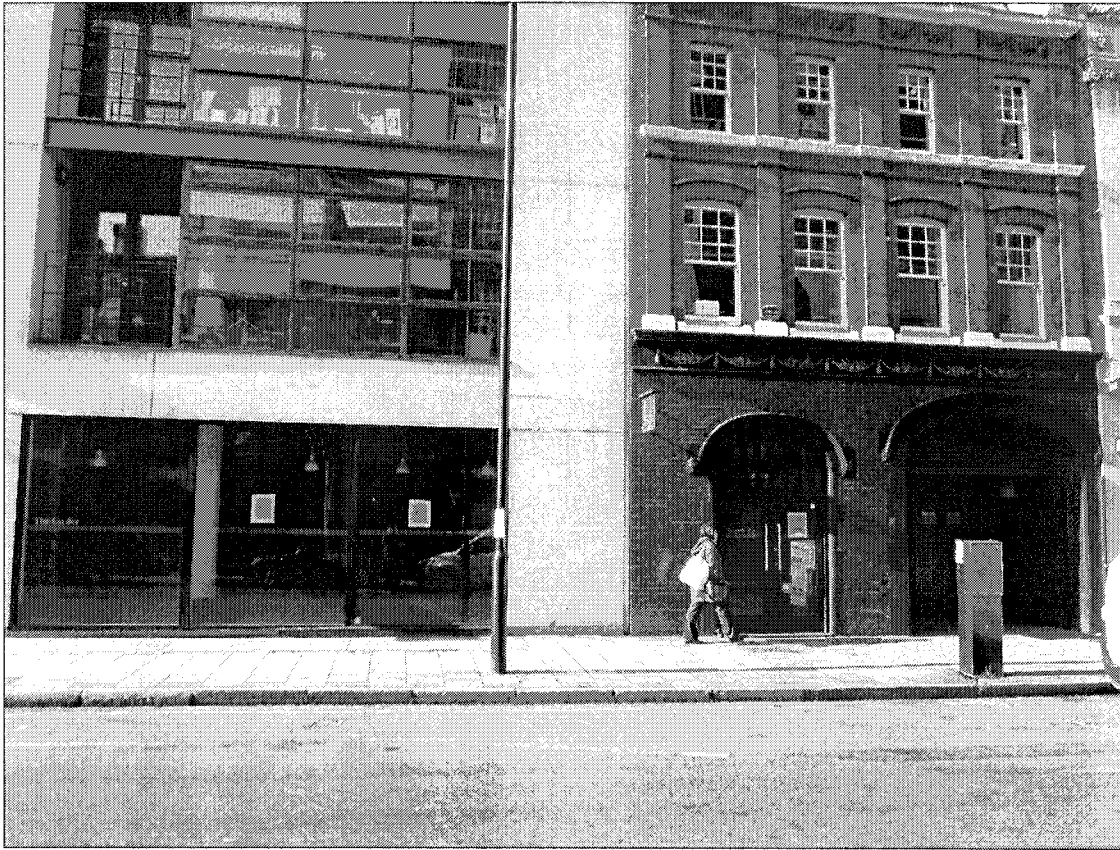
Front elevation (east facing) of application site viewed from opposite footpath.
