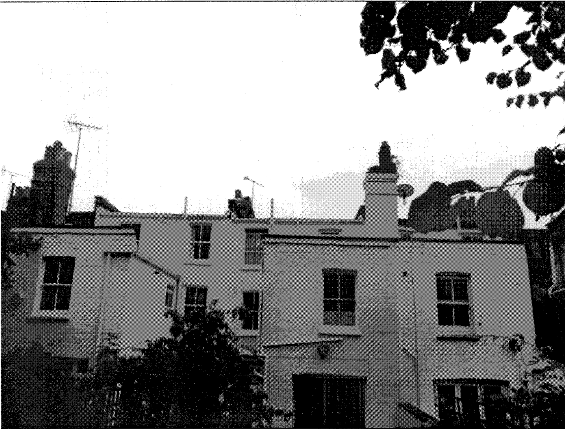
View from rear garden of 95 Harberton Road.
