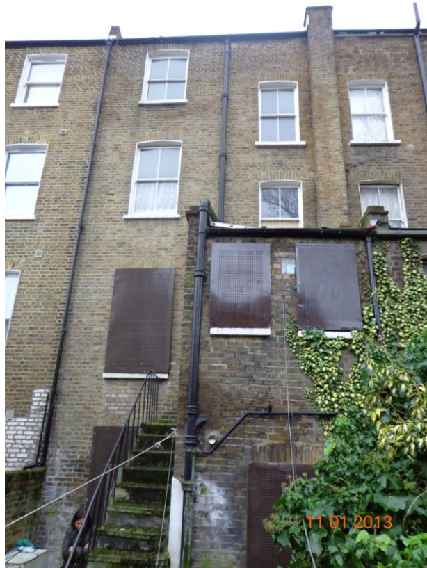
Rear Elevation of 15 Tabley Road
