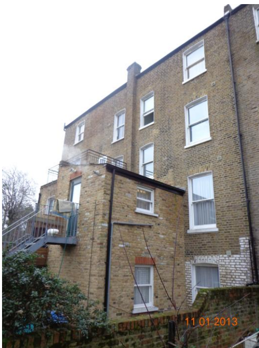
View to the rear of elevation of 13 and 17 Tabley Road
