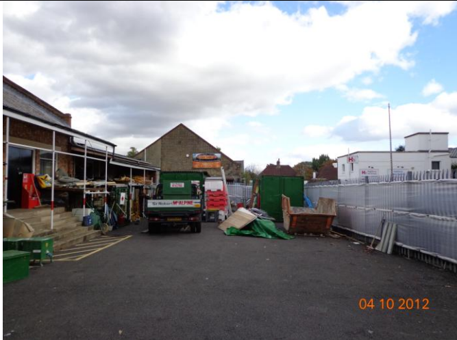
EXISTING YARD TO REAR OF THE COACH HOUSE. BUILDINGS TO BE DEMOLISHED ARE SITED TO THE LEFT.
