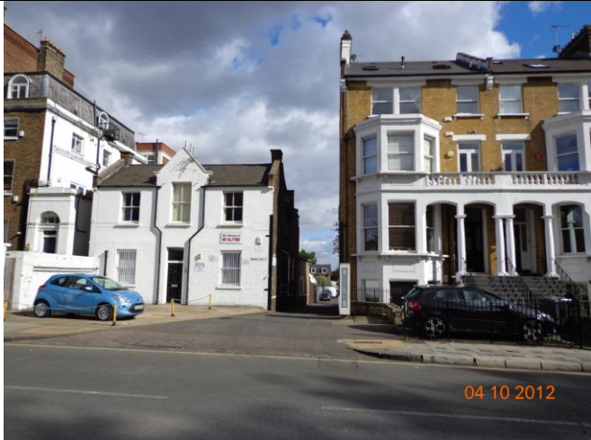
ACCESS BETWEEN NO'S 56 & 58 Highbury Grove.
