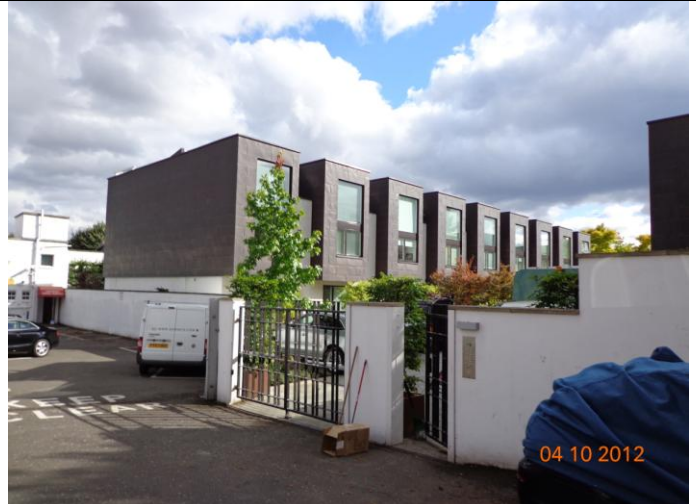
GATED CONTEMPORARY DEVELOPMENT IMMEDIATELY TO THE SOUTH (NO'S 6 – 32 MELODY LANE).
