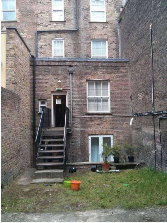
Towards rear elevation of building.
