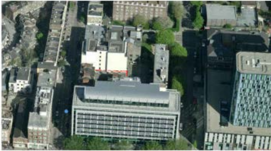
Photo 1: Aerial view from the south
