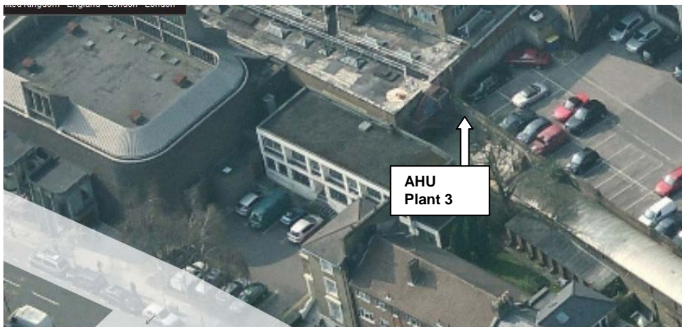
Photo 3: Aerial photography showing proposed position of the air-handling unit in the yard
