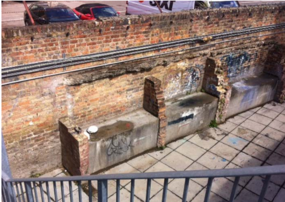
Photo 6: Positioning of AHU 3 in the yard.
