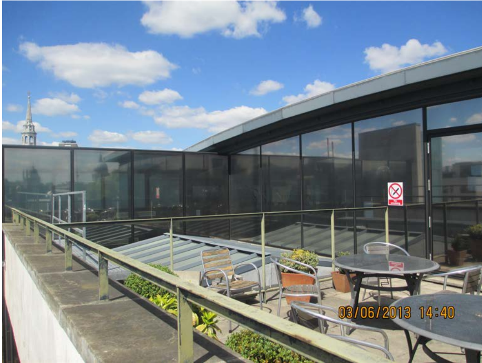
Photo 3: View of location of existing fourth floor terrace
