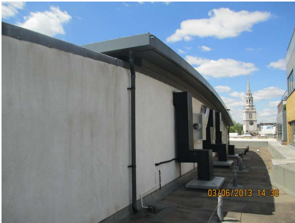
Photo 4: Eastern elevation facing One Britton Street
