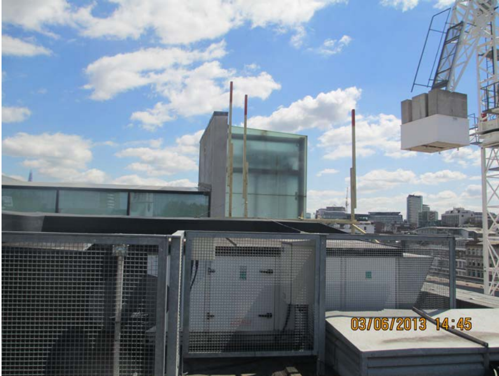
Photo 5: View of existing plant looking south.
