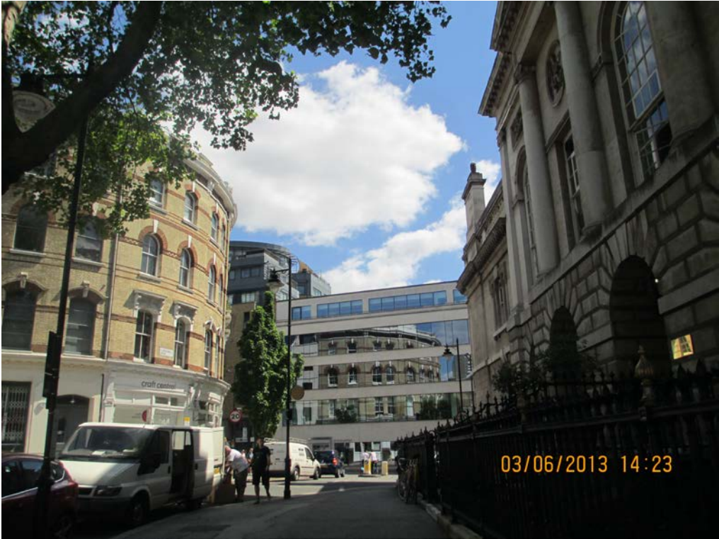
Photo 1: View of application site from Clerkenwell Green.
