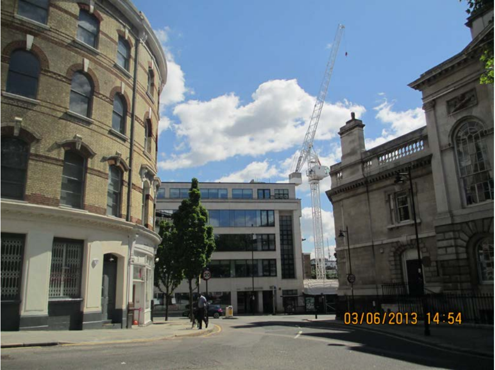
Photo 2: View of application site from Clerkenwell Green
