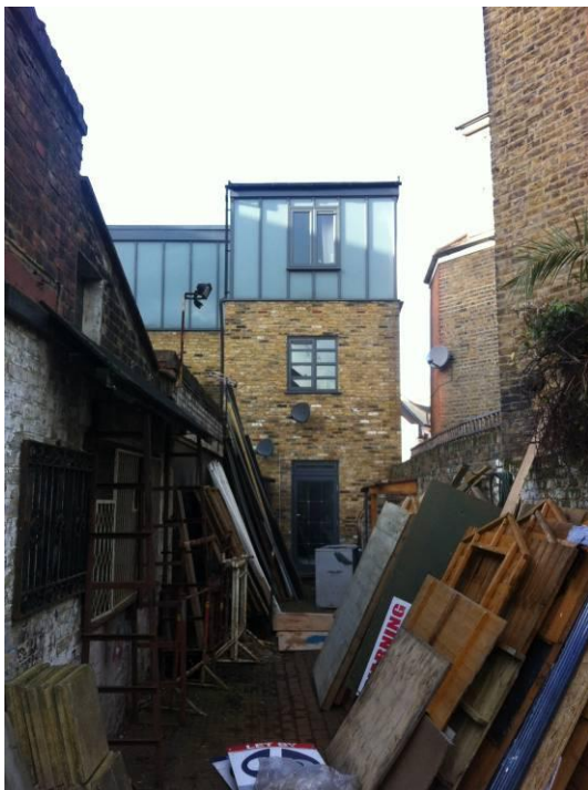
Photo 2: Towards rear of Mews. Building to end of mews is offices.
