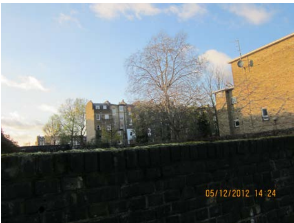
Photos 5 & 6 View of application site from the rear
