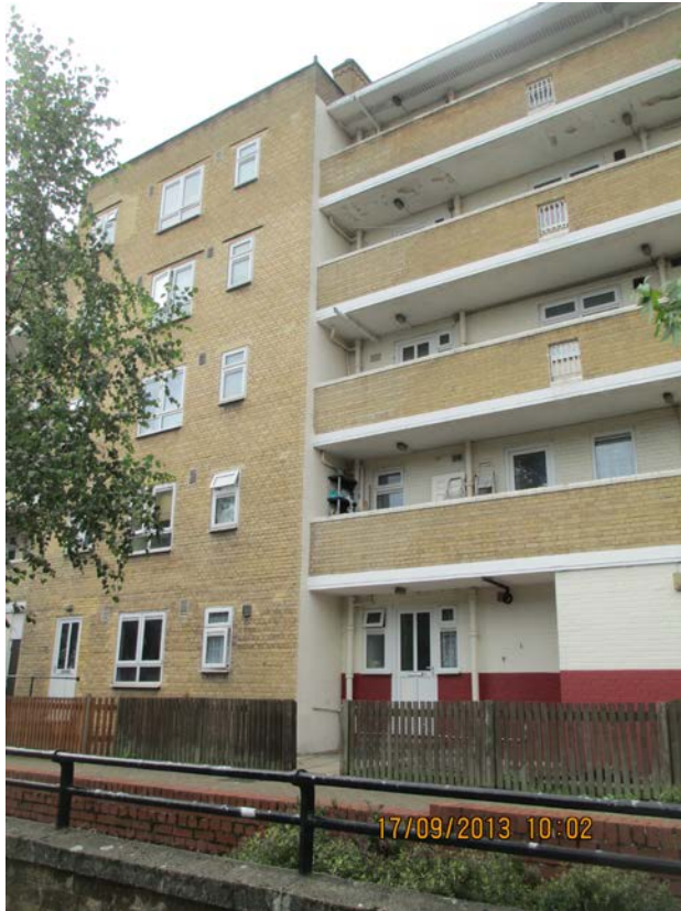
5. The external walkways
