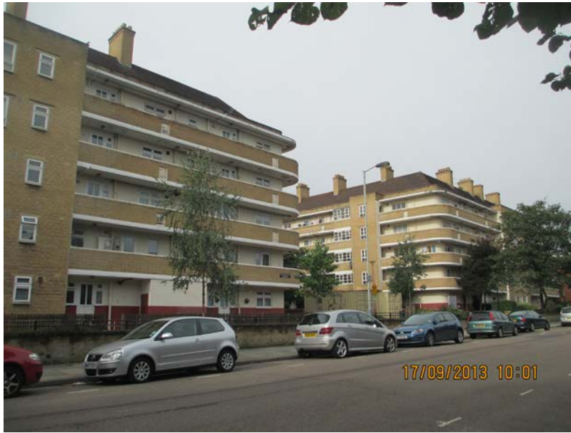
3. Buckhurst House (foreground) and Coombe House
