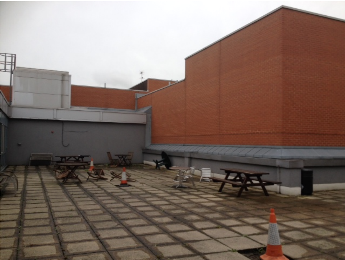
Photograph 3: The site looking south east.
