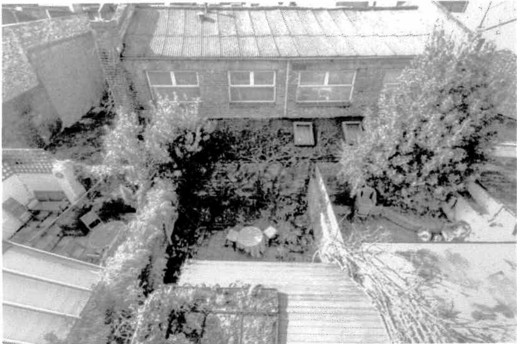
Photo 1. Ground floor extension at the rear of No. 88/90 Holloway Roa
