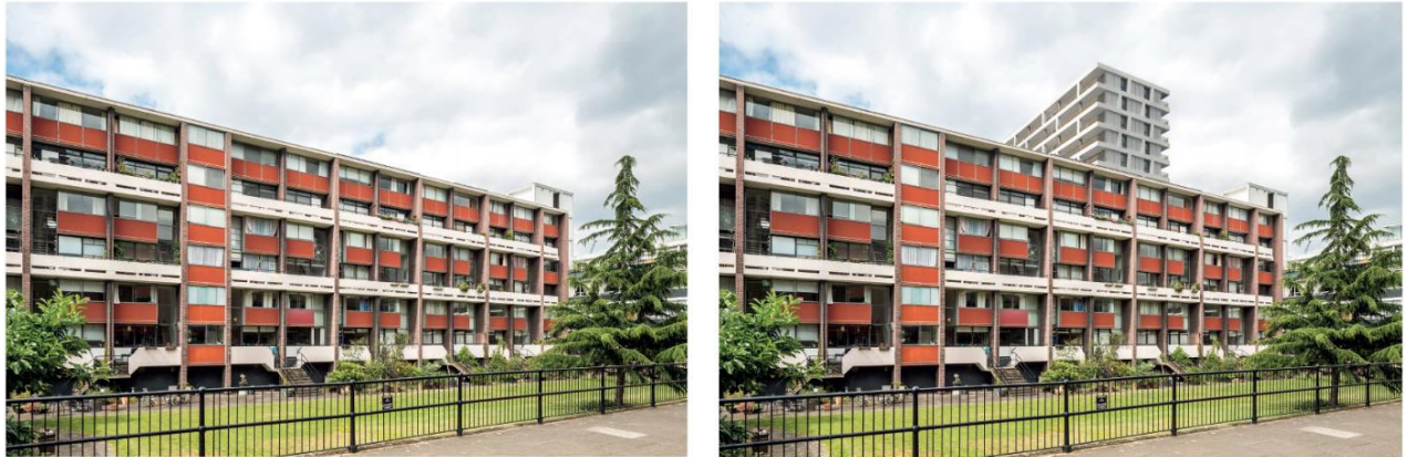
View 10 – Golden Lane Estate looking north-east towards Basterfield House
