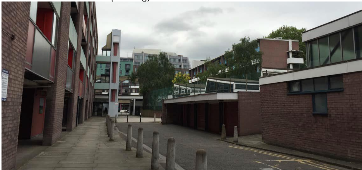
Basterfield Service Road (Existing)
