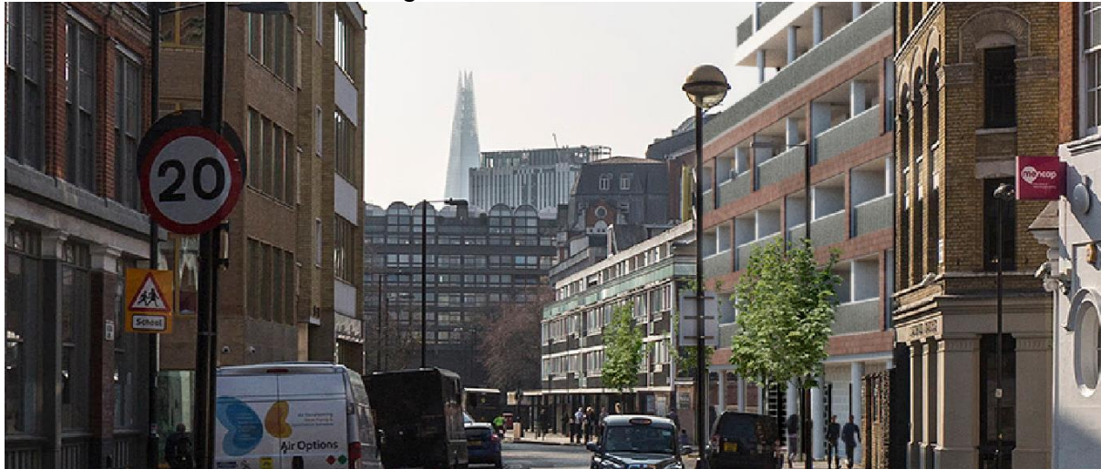
Podium on Golden Lane frontage
