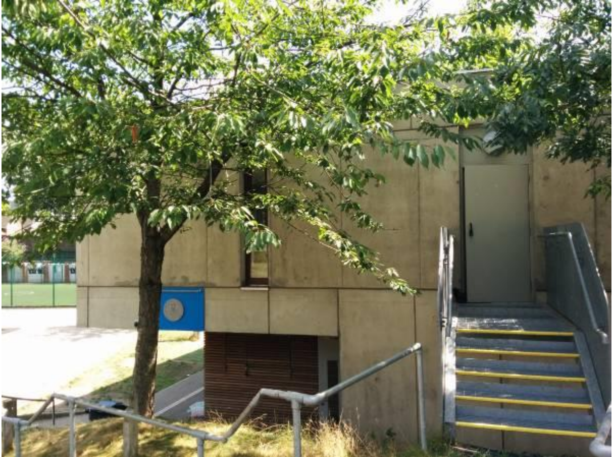
Photo 3 – Existing tree and interface location of fence with existing building.
