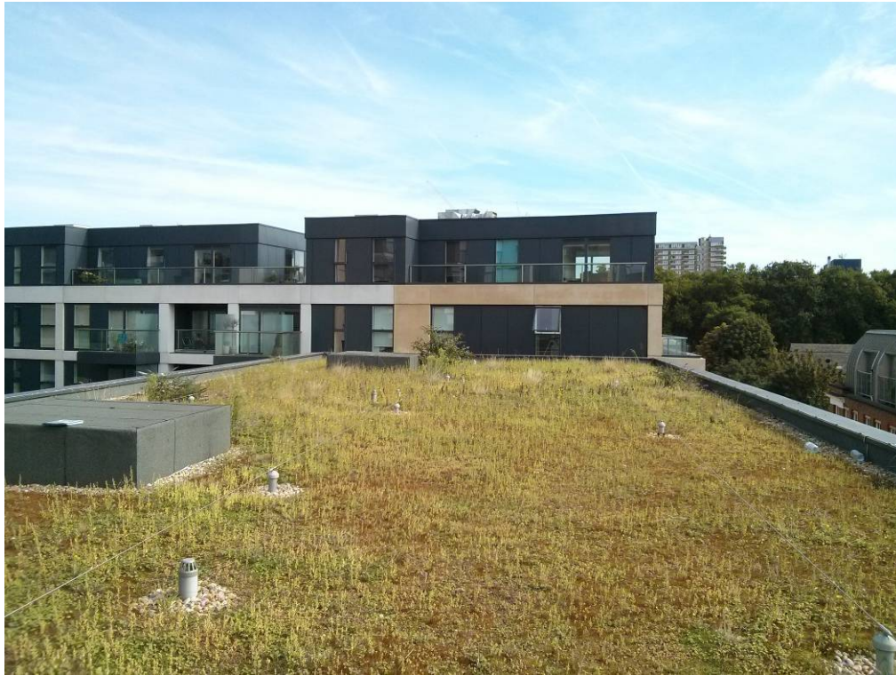
Photo 1: View east of existing roof space.
