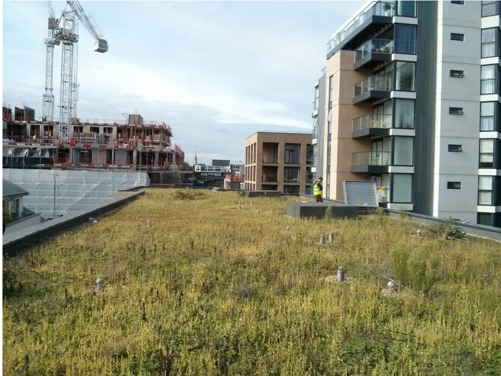
Photo 2: View west of existing roof space.
