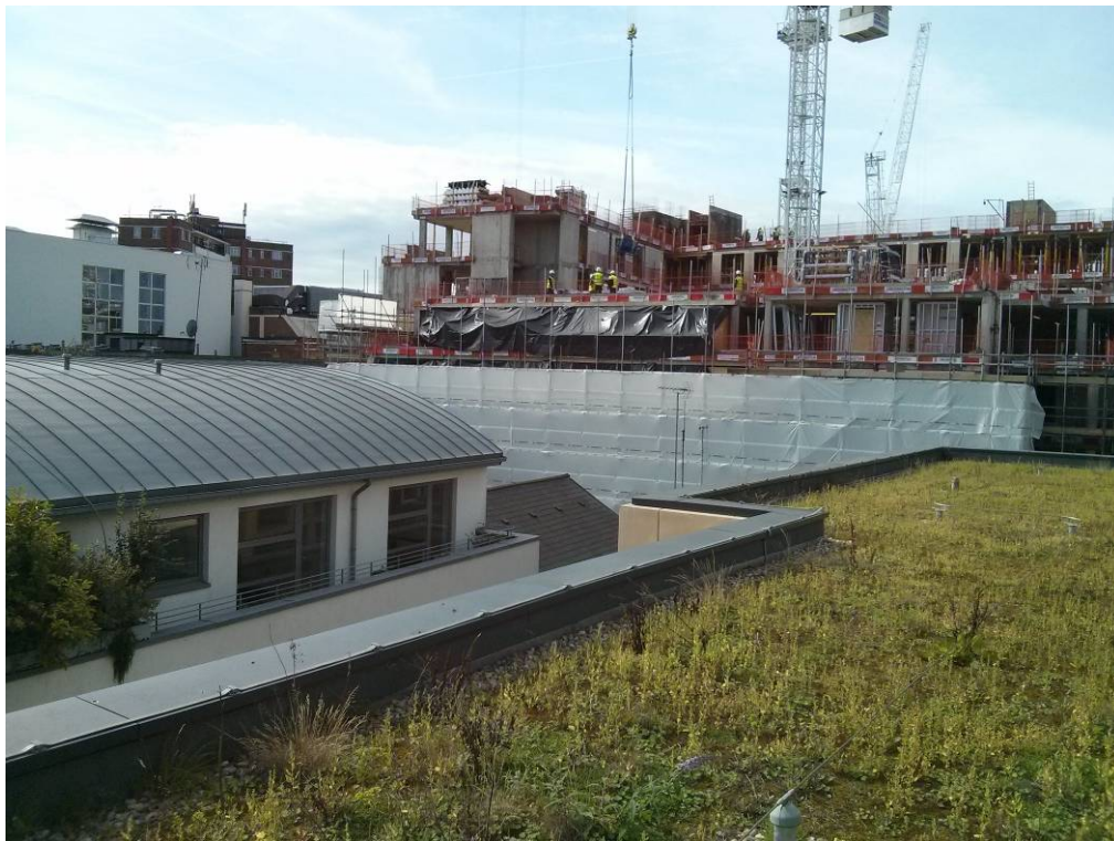
Photo 4: Looking south towards Pear Tree Street.
