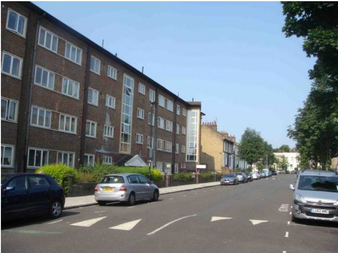
Figure 68 Wells Court (centre-left of picture), which is located on Queen Margaret's Grove was constructed during the 1950s.
