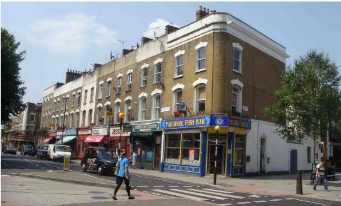
Figure 51 Numbers 125 to 141 (odd) Newington Green Road. Note that this group was constructed during the 1860s.
