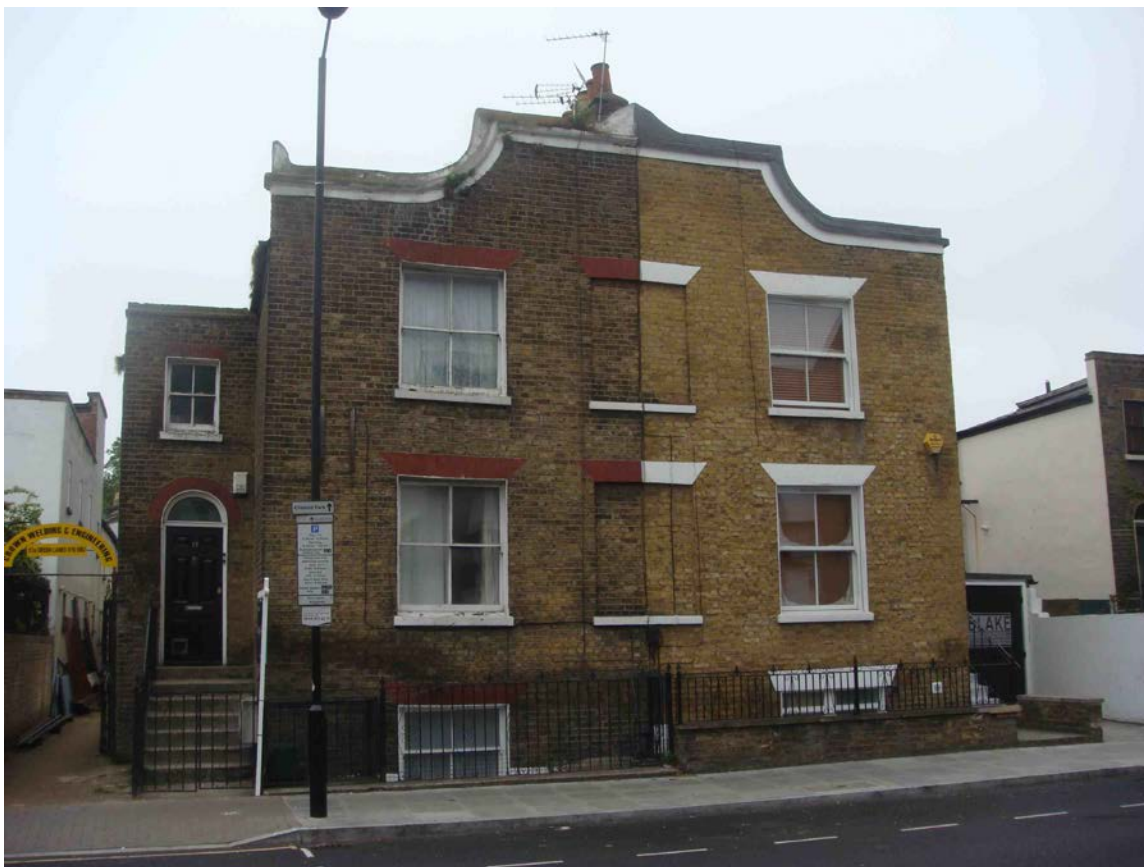
Figure 40 Numbers 53 and 55 Green Lanes. Note that the original form of this pair is unaltered. The boundary wall and railings date from the late twentieth century. The two-over-two sash windows are likely mid nineteenth century replacements
