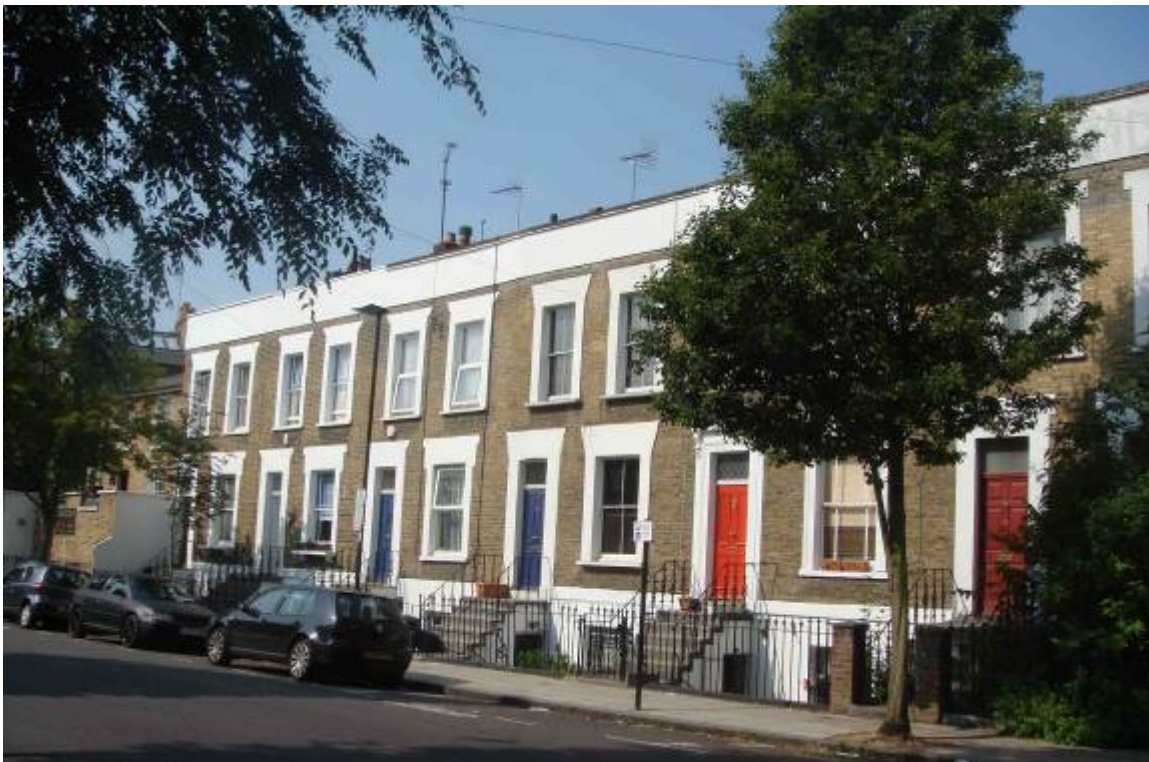
Figure 48 Numbers 15 to 17 (odd) Wolsley Road. Note that these buildings date from the mid nineteenth century.
