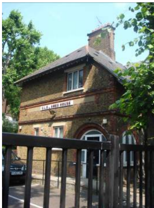
Figure 59 C.L.R James House formerly known as 'Founders Lodge' as part of the Mildmay Hospital and Compound complex. Note that this building dates from the late nineteenth century
