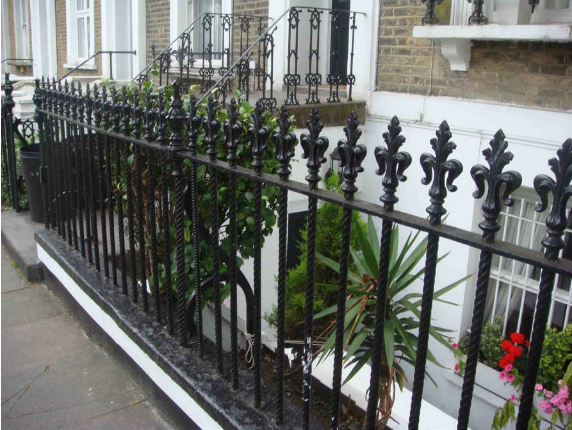
Figure 73 Historic nineteenth century railings located on Mildmay Road
