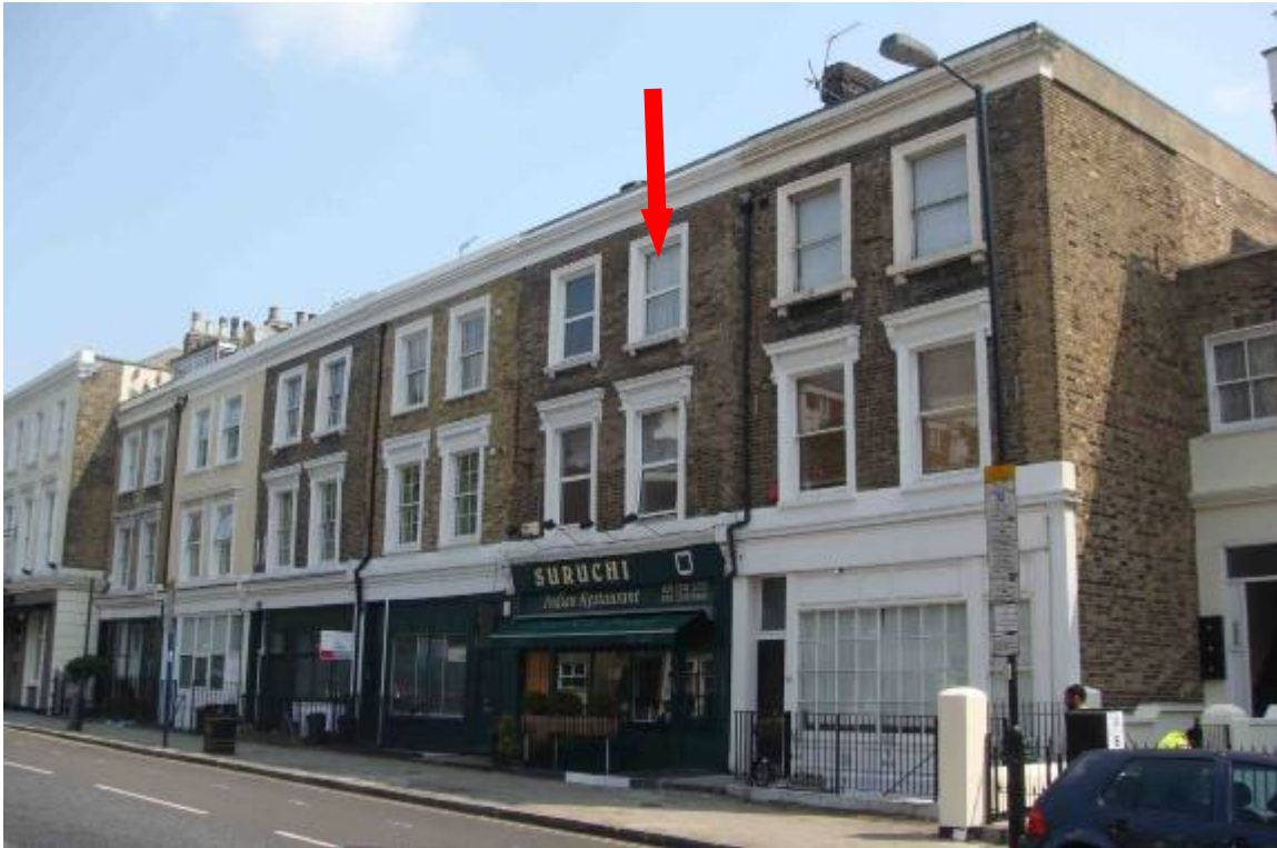
Figure 49 Numbers 80 (left of picture) to 90 (right) Mildmay Park. Note the range of window types within this terrace, which include mid nineteenth century six-over-six timber sashes (with slim side lights) and more recent uPVC replacements (example arrowed).
