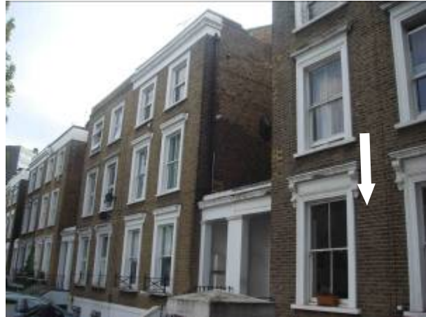
Figure 44 Typical two-over-two sash window to a building on Mildmay Park. Note the original pilasters to window surrounds and decorative hoods with console brackets (arrowed) at ground level
