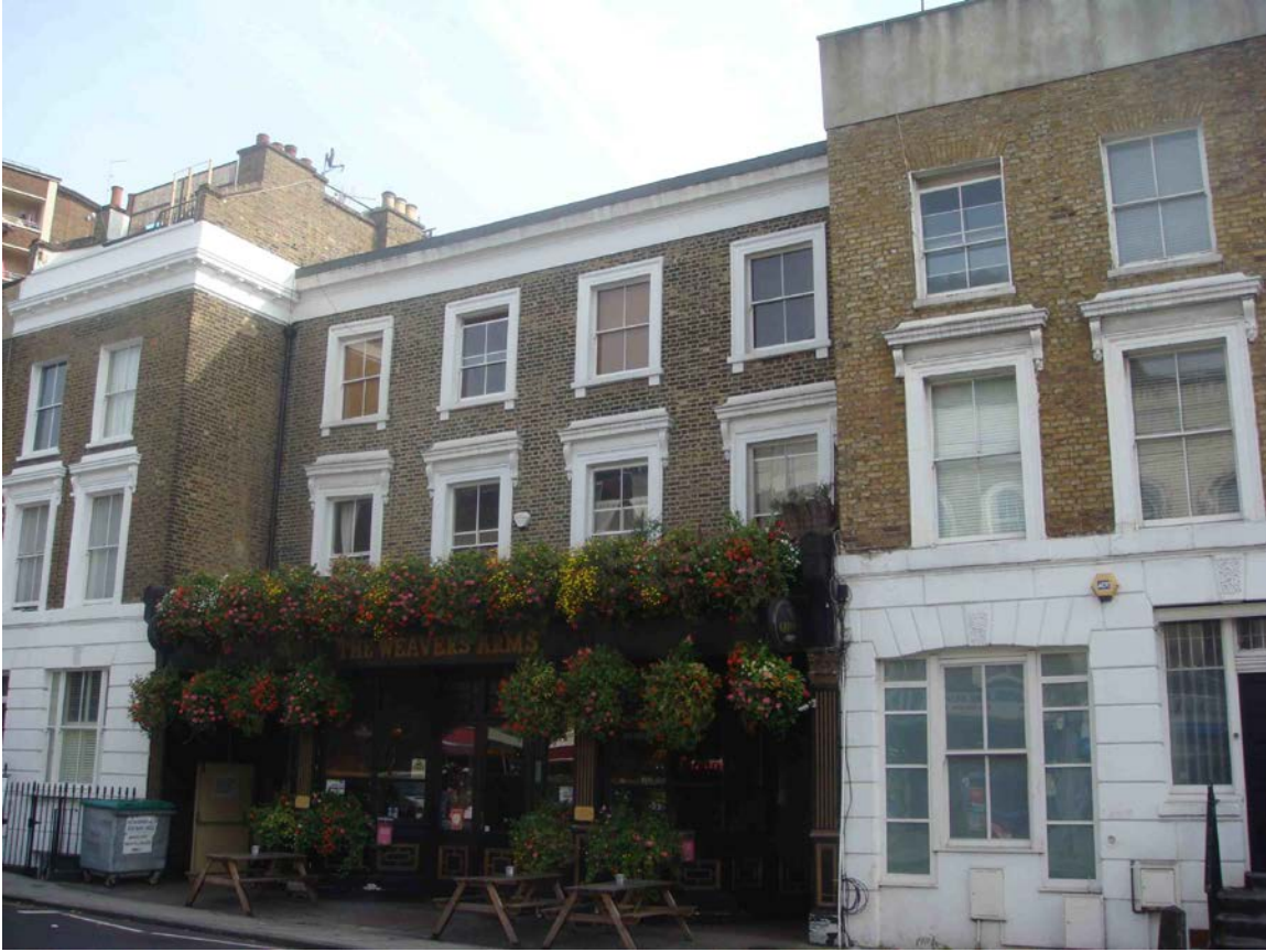
Figure 70 The Weavers Arms located at number 98 Newington Green Road. Note the timber frontage.
