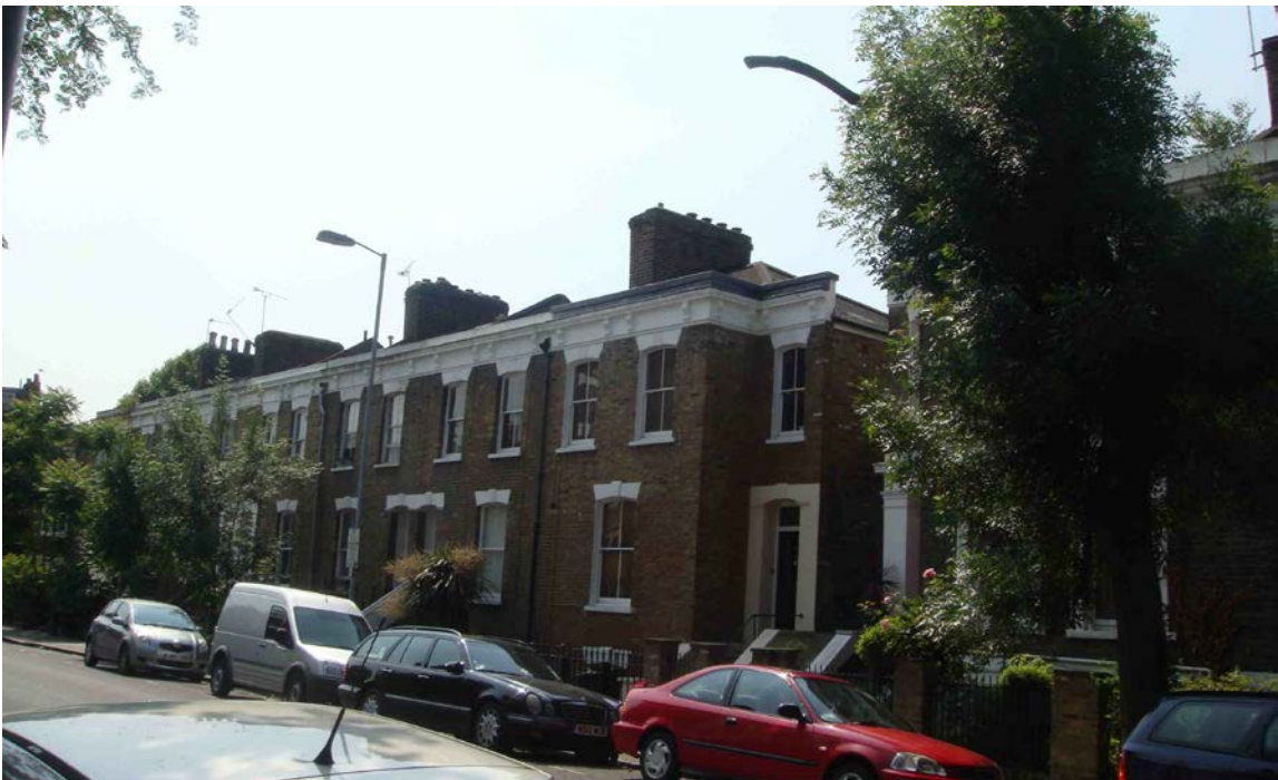
Figure 57 Part of two-storey terrace group located at numbers 21 to 33 (odd) Mildmay Road
