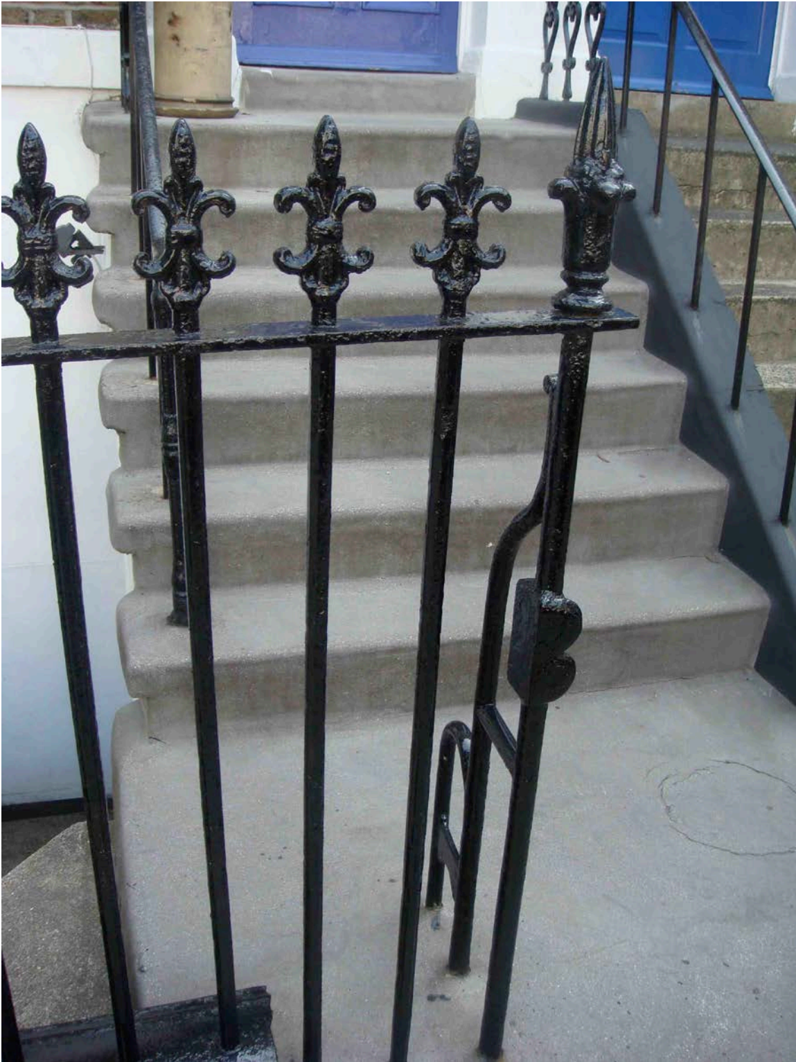
Figure 72 Mid nineteenth century boundary railing detail on Wolsley Road
