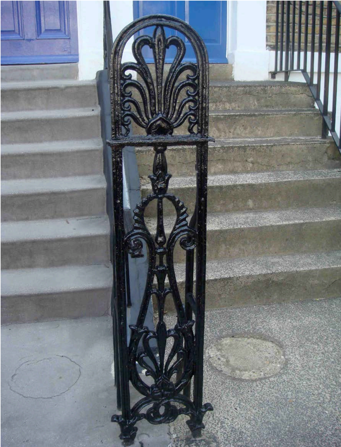
Figure 71 Mid nineteenth century rail and gate post detail on Wolsley Road
