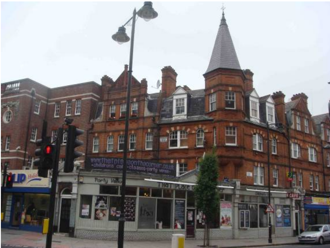
Figure 58 Newington Green Mansions, which occupies a prominent corner site on the northwest corner of Newington Green. Note the spirelet, which is a notable landmark feature in the area.
