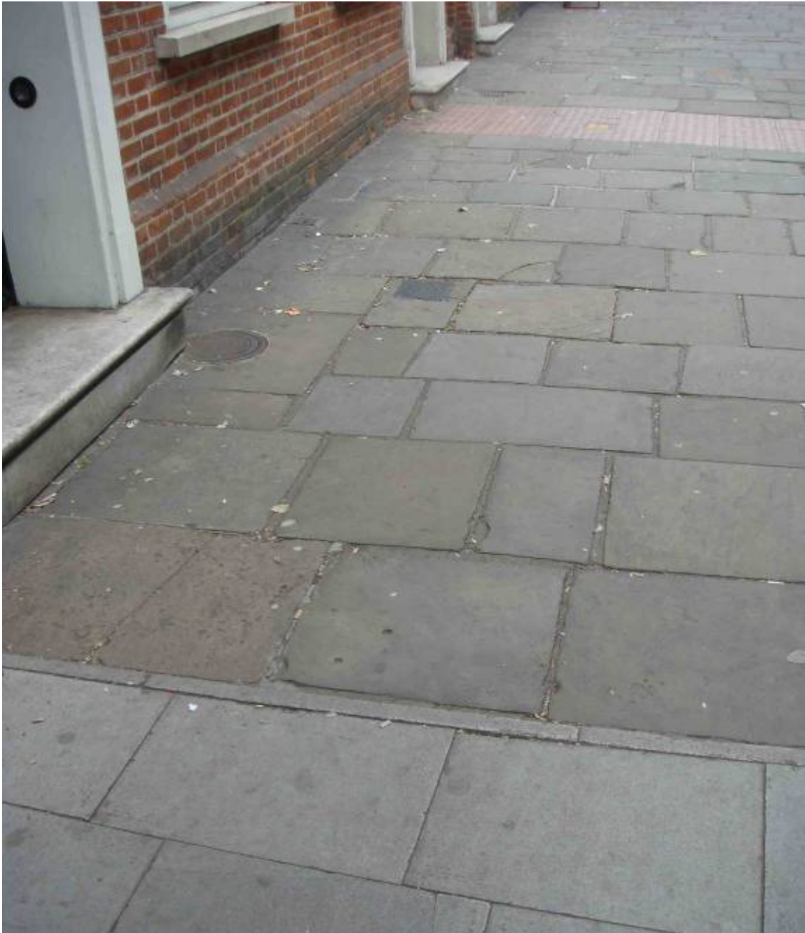
Figure 75 Historic York stone paving (centre top of picture) to the front of numbers 52 to 55 Newington Green. Note the contrast with the concrete paving (bottom of picture)
