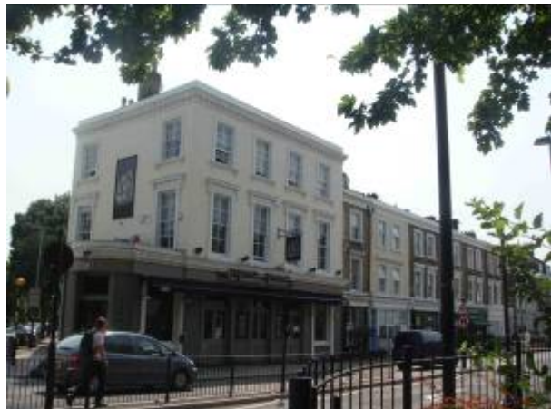
Figure 27 Numbers 80 (far right of picture) to 92 (centre left) Mildmay Park. Note that this terrace group adjoins the southeast corner of Newington Green
