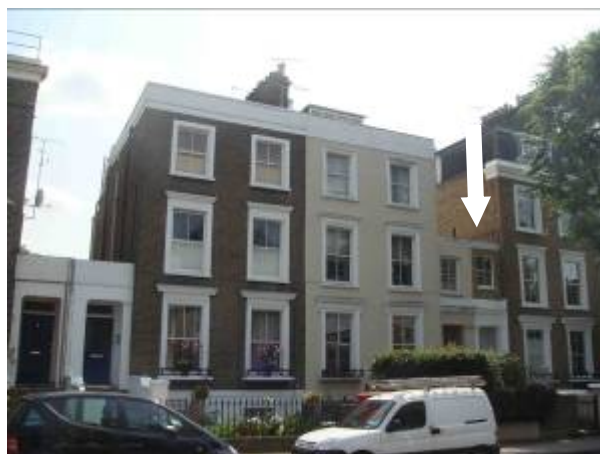
Figure 42 Numbers 70 (far right of picture) to 74 (centre left) Mildmay Park. Note the original single storey entrance porch to number 74 and the altered porches at numbers 70 and 72 (arrowed)
