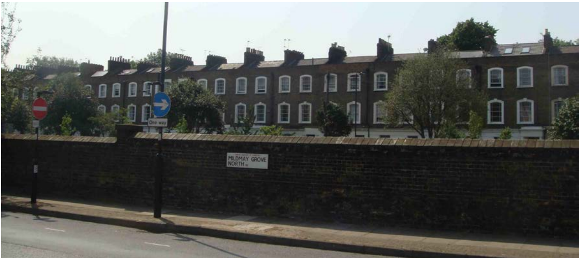
Figure 55 Pitched roofs set behind raised parapets to a terrace group located on Mildmay Grove South. Note picture is taken from Mildmay Grove North
