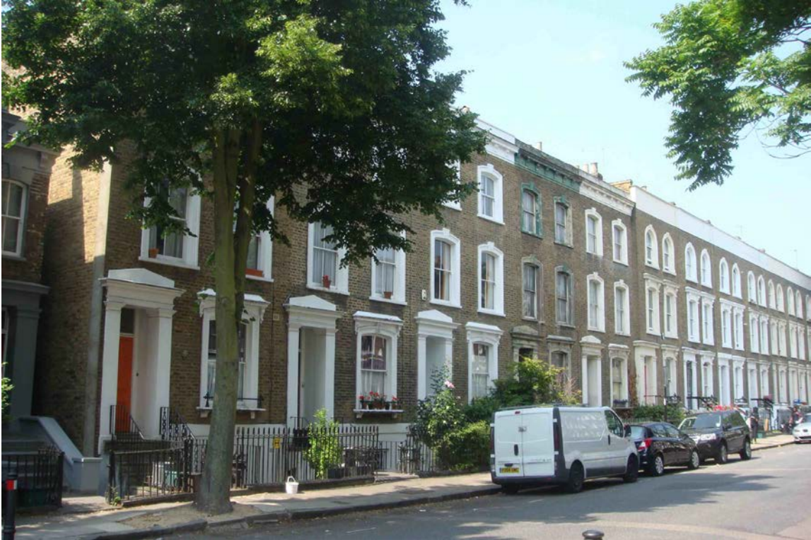
Figure 56 Eastern part of terrace located at 59 to 119 Mildmay Road.
