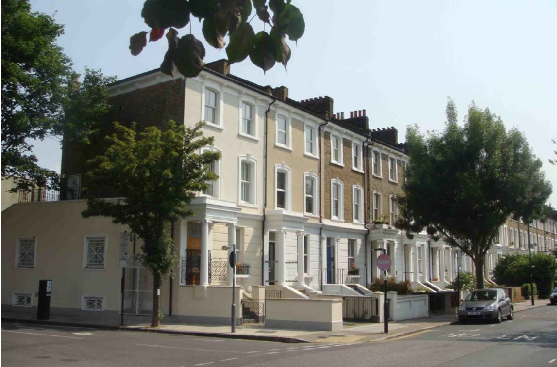
Figure 54 Western end of terrace group located at numbers 51 to 109 Mildmay Grove North
