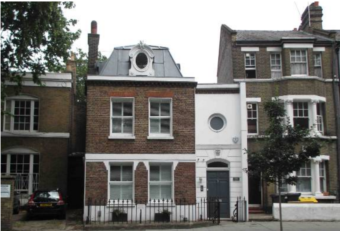
Figure 39 Number 30 Newington Green (centre of picture). Note that this building dates from the early nineteenth century with later nineteenth century alterations, including replacement sash windows
