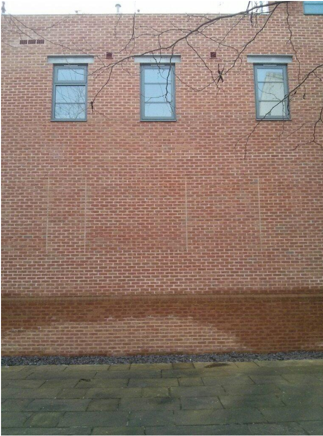
Photo 1: North elevation where windows are to be installed.
