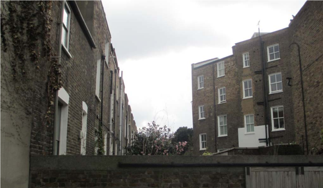
Rear elevation and gap between properties
