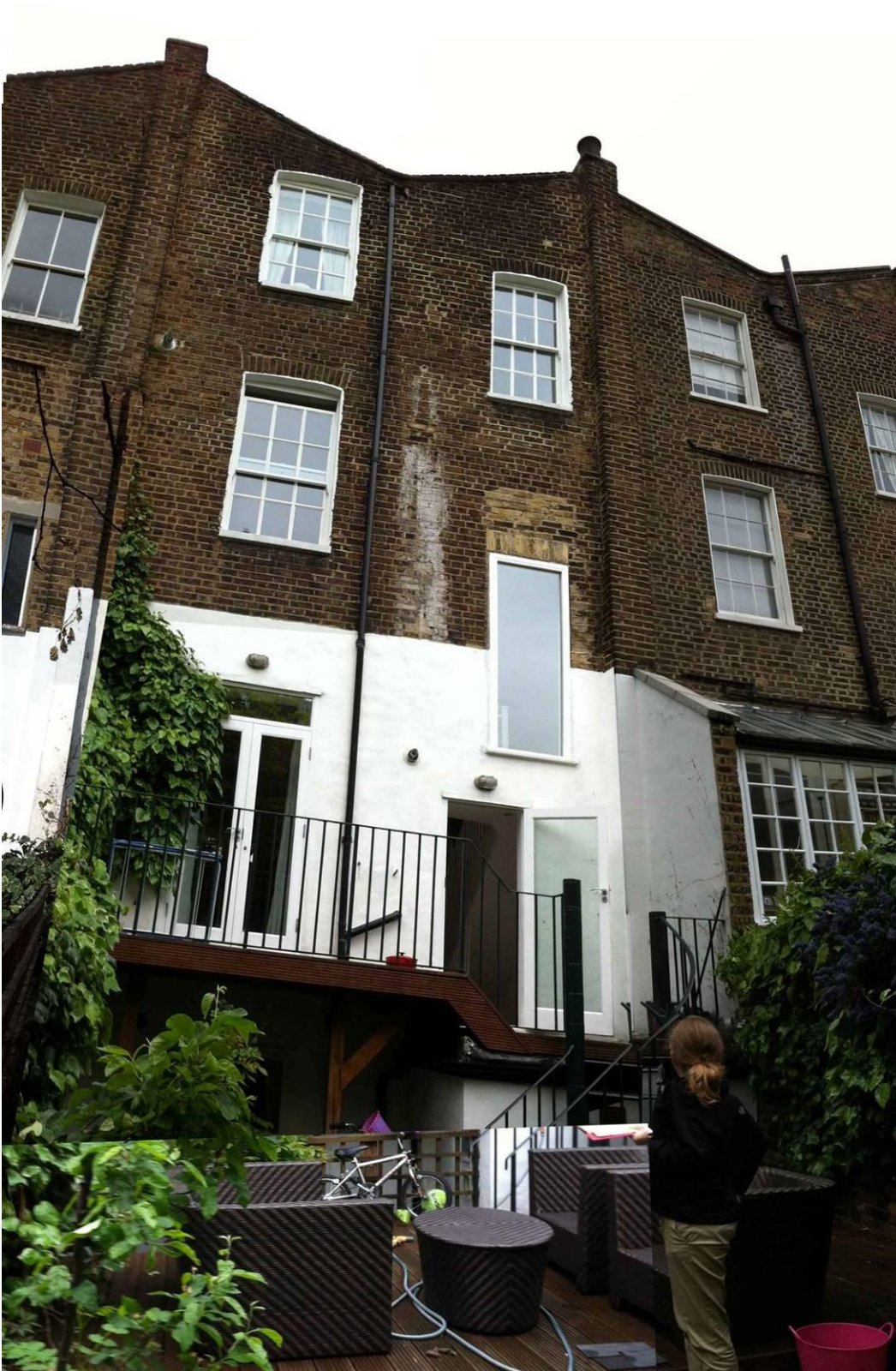
Photo 1: Rear of elevation of property. NB: Railings and decking have been removed.
