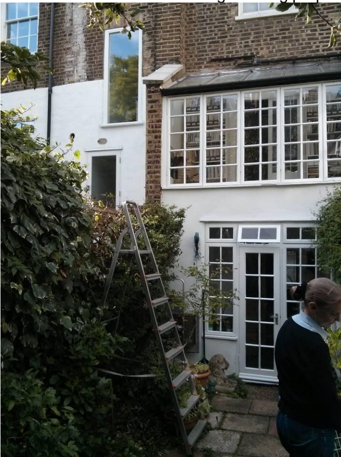
Photo 3: Rear elevation of neighbouring property at no. 18
