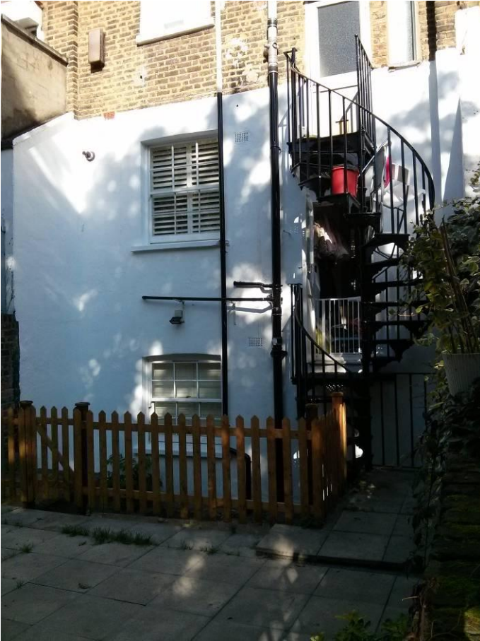
Photo 2: Rear elevation of neighbouring property at no. 20
