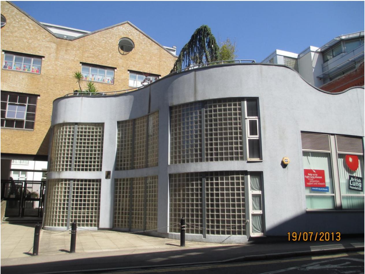
2. View of front elevation of site
