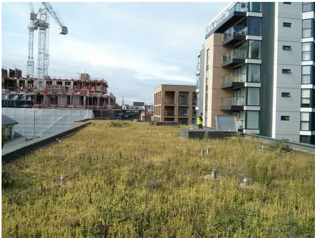
Photo 2: View west of existing roof space.
