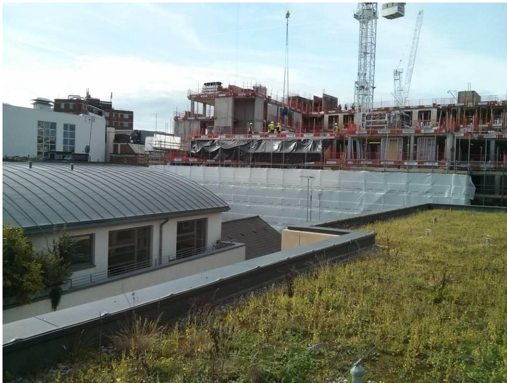
Photo 4: Looking south towards Pear Tree Street.
