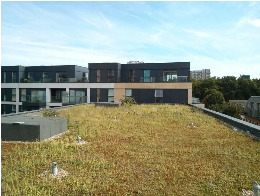
Photo 1: View east of existing roof space.
