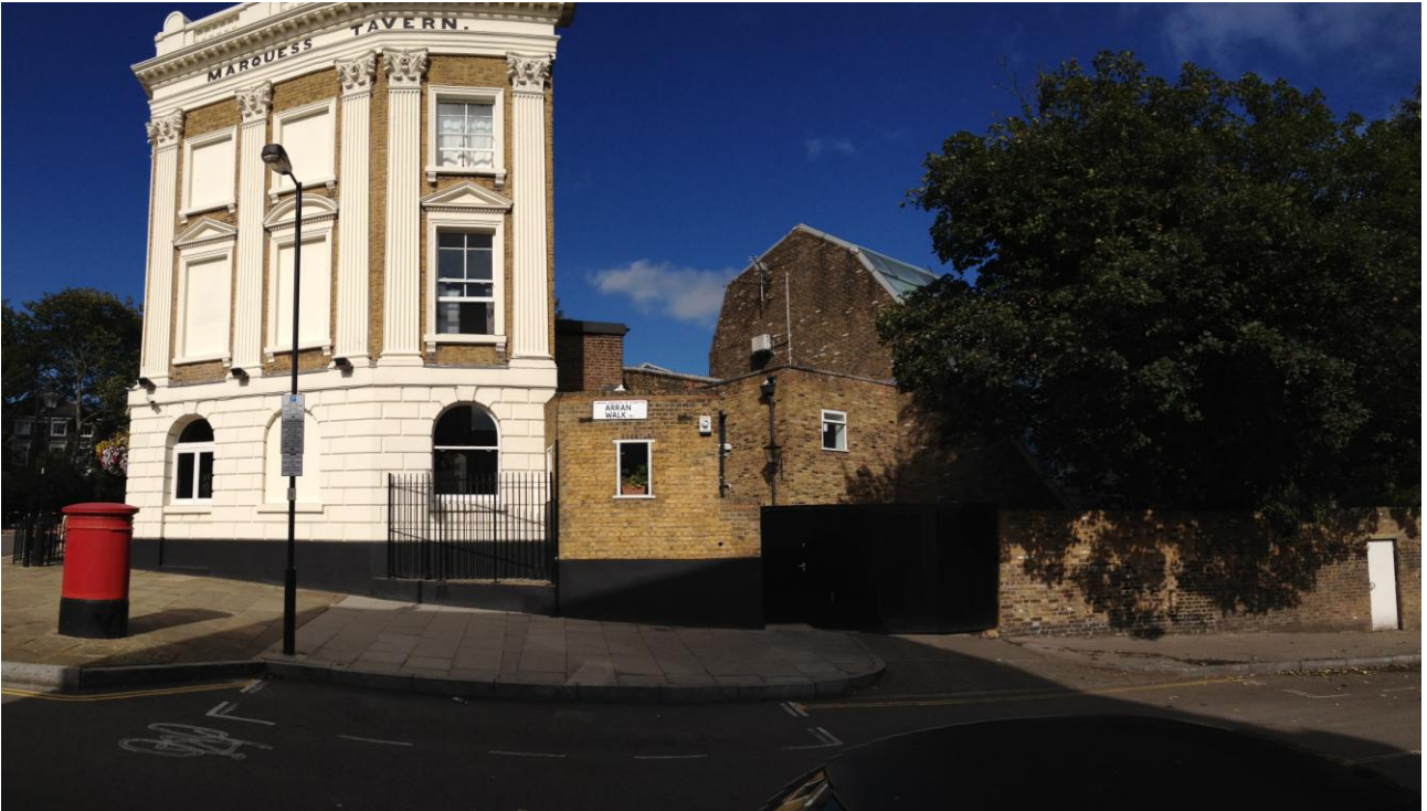
Photo 1: Southern elevation of host site, viewed from Arran Walk
