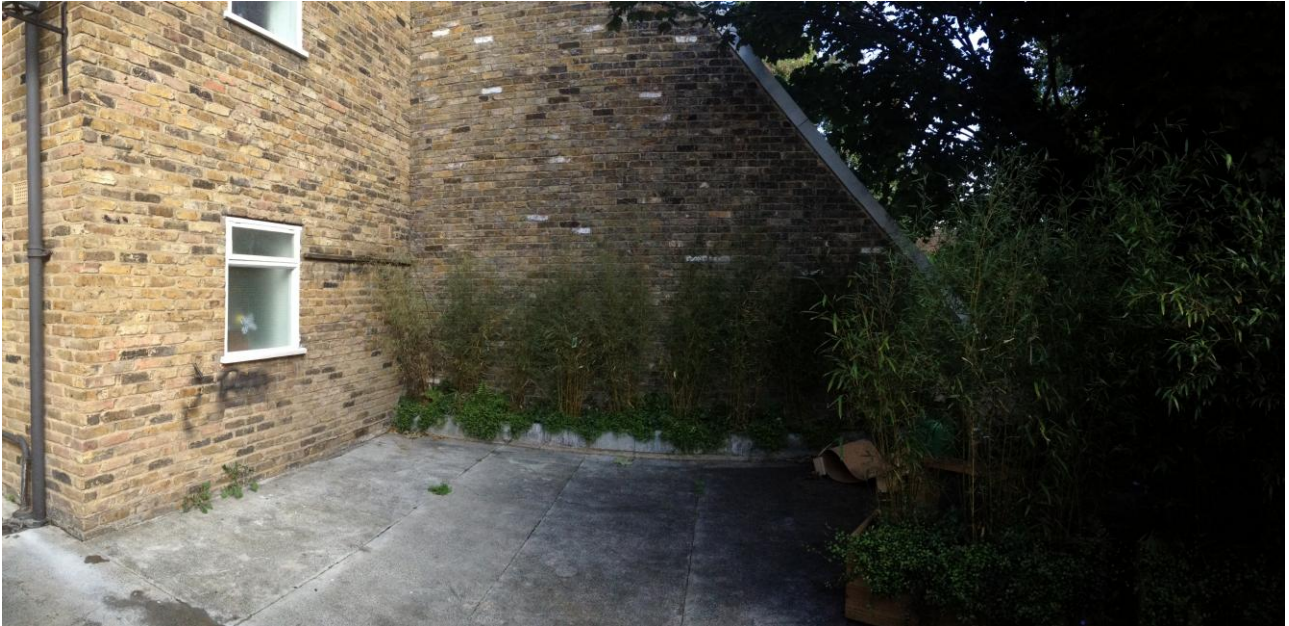
Photo 3: Location of proposed works, rear yard facing east.
