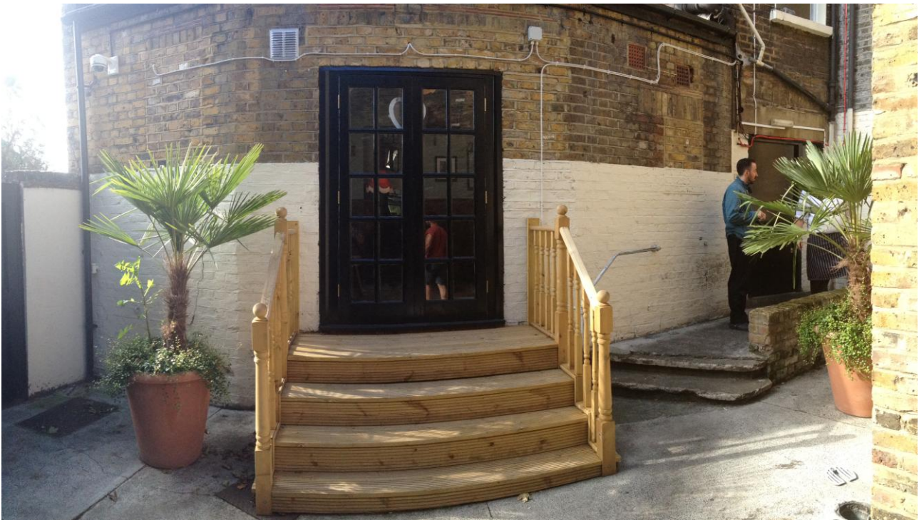
Photo 4: Eastern elevation of Marquess Tavern, stairs leading to rear yard from dining area
