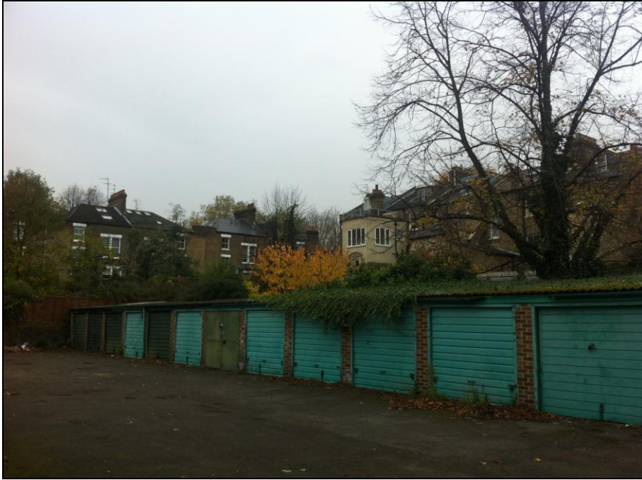
View of proposed garages to be demolished.
