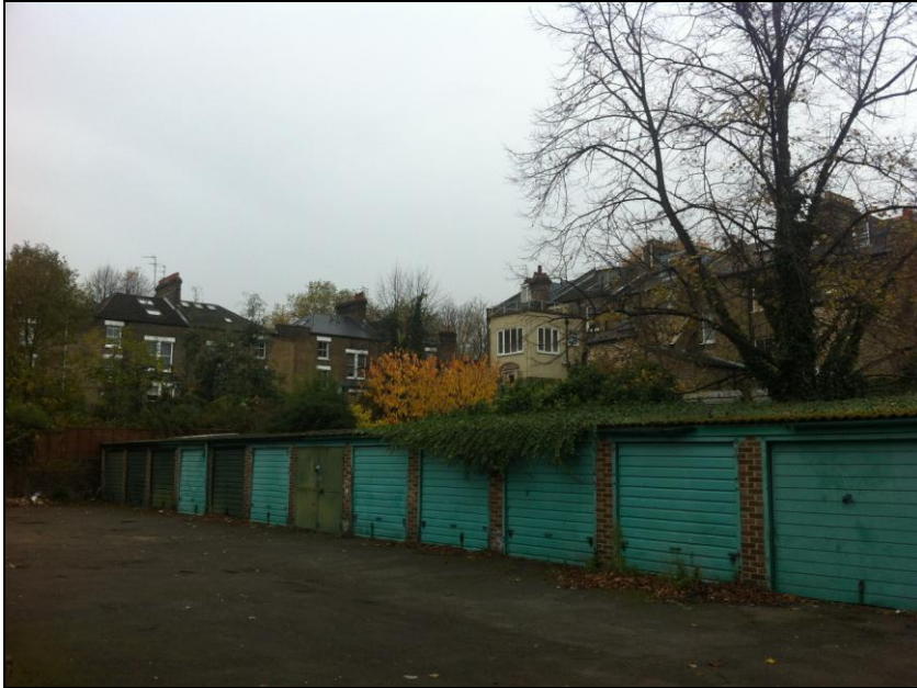
View of proposed garages to be demolished.
