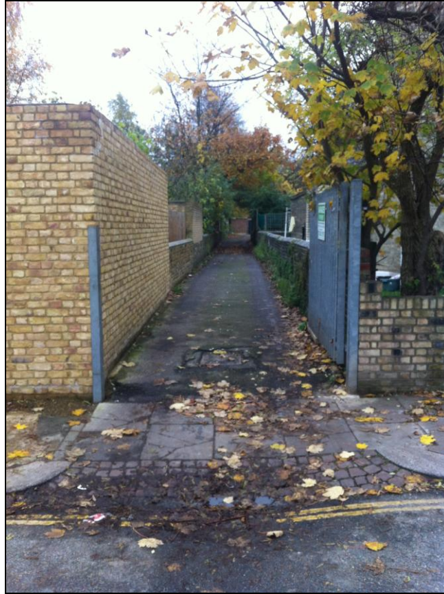
View of the main vehicular access to the site from Cardozo Road.
