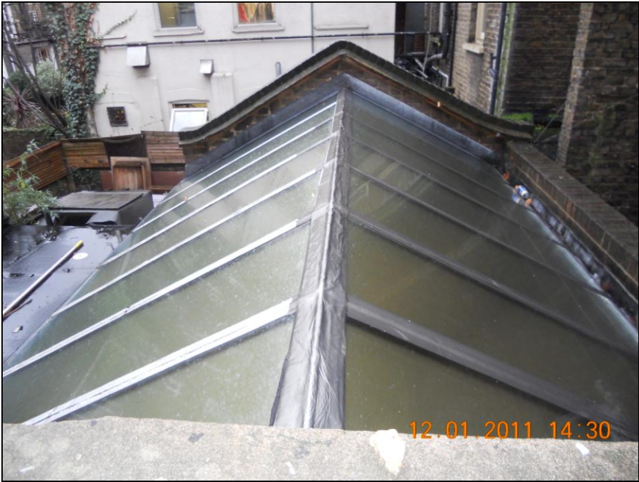
Photo 3: View of existing rear roof slope
