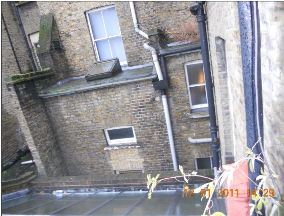
Photo 4: View of rear elevation of 263 Upper Street
