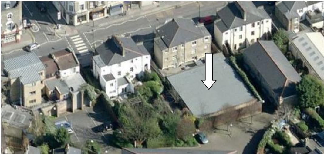
Photo 2: Aerial photograph of site
