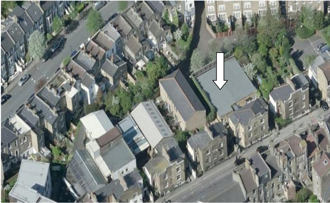
Photo 1: Aerial photograph of site
