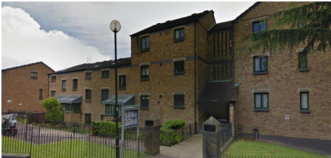
3. View of the site from Mount View Road
