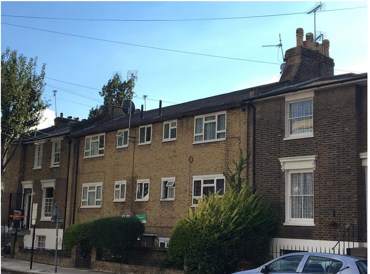
Image 1: Photograph of front of site showing roof
