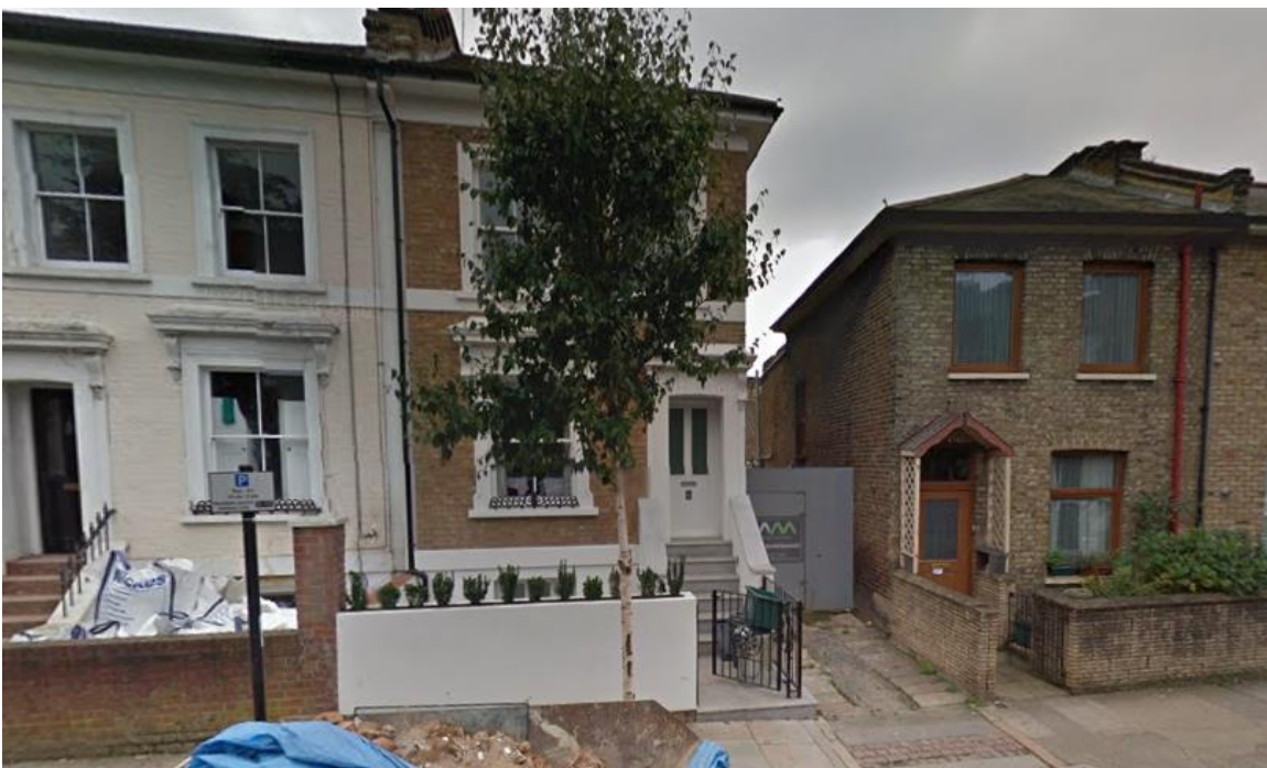
Image 1 – Frontage of No. 6 Shaftesbury Road with access to application site between No. 4 and 6 Shaftesbury Road
