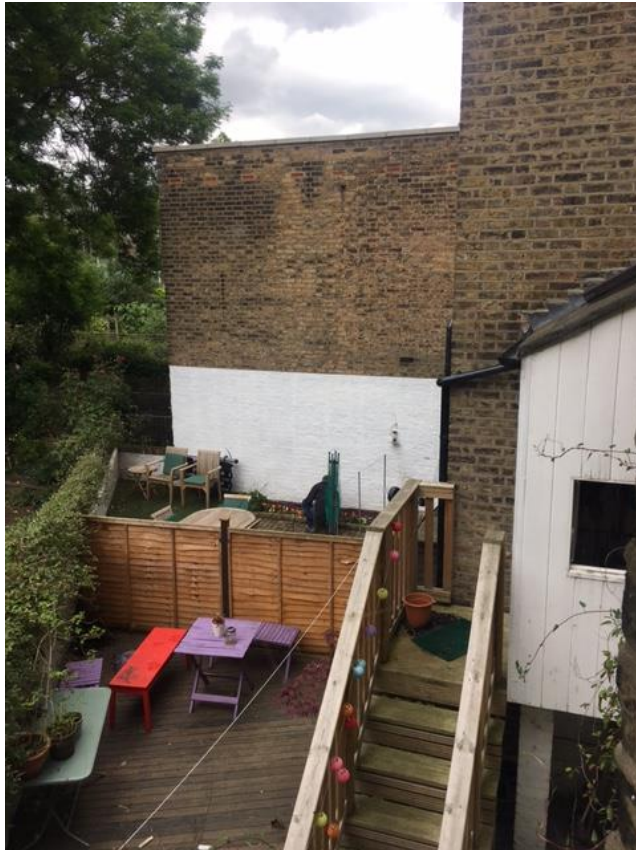
Image 2: View of existing site from neighbouring property
