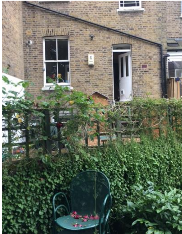
Image 4: Existing rear elevation taken from back of garden 60 Huddleston Road
