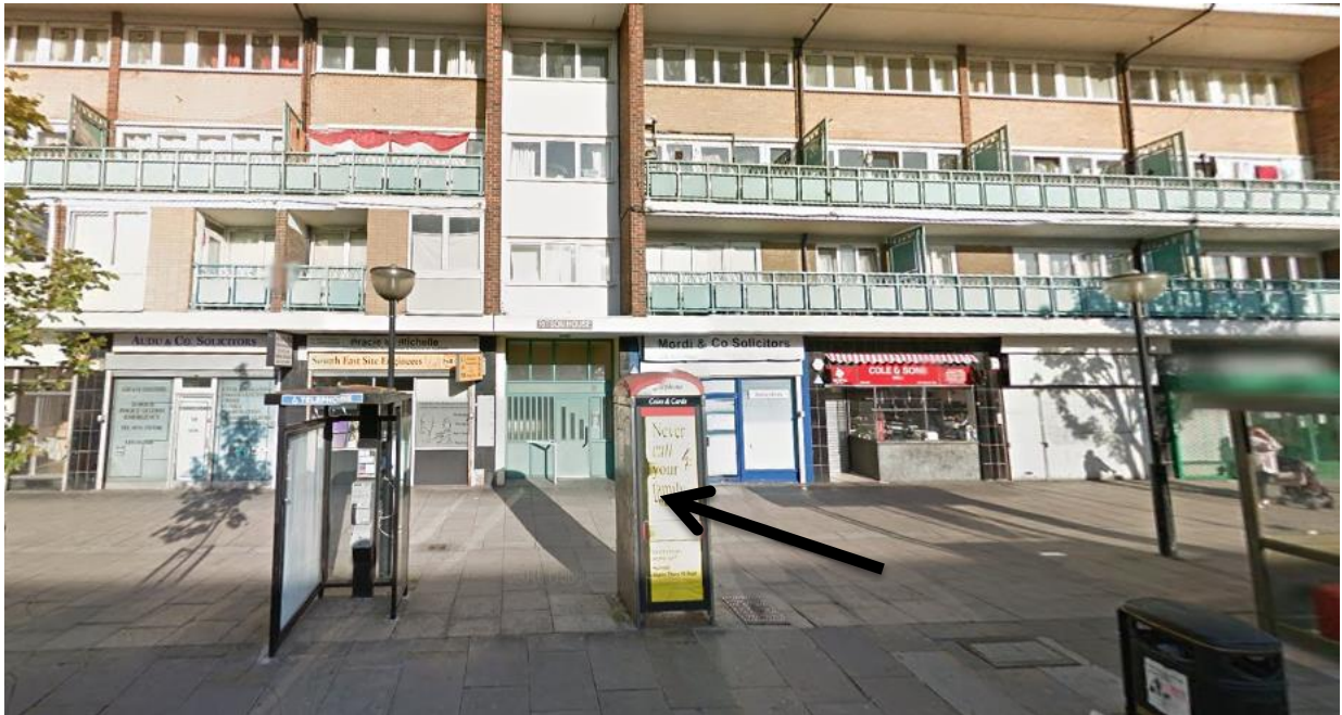
Image 1: View of the site
