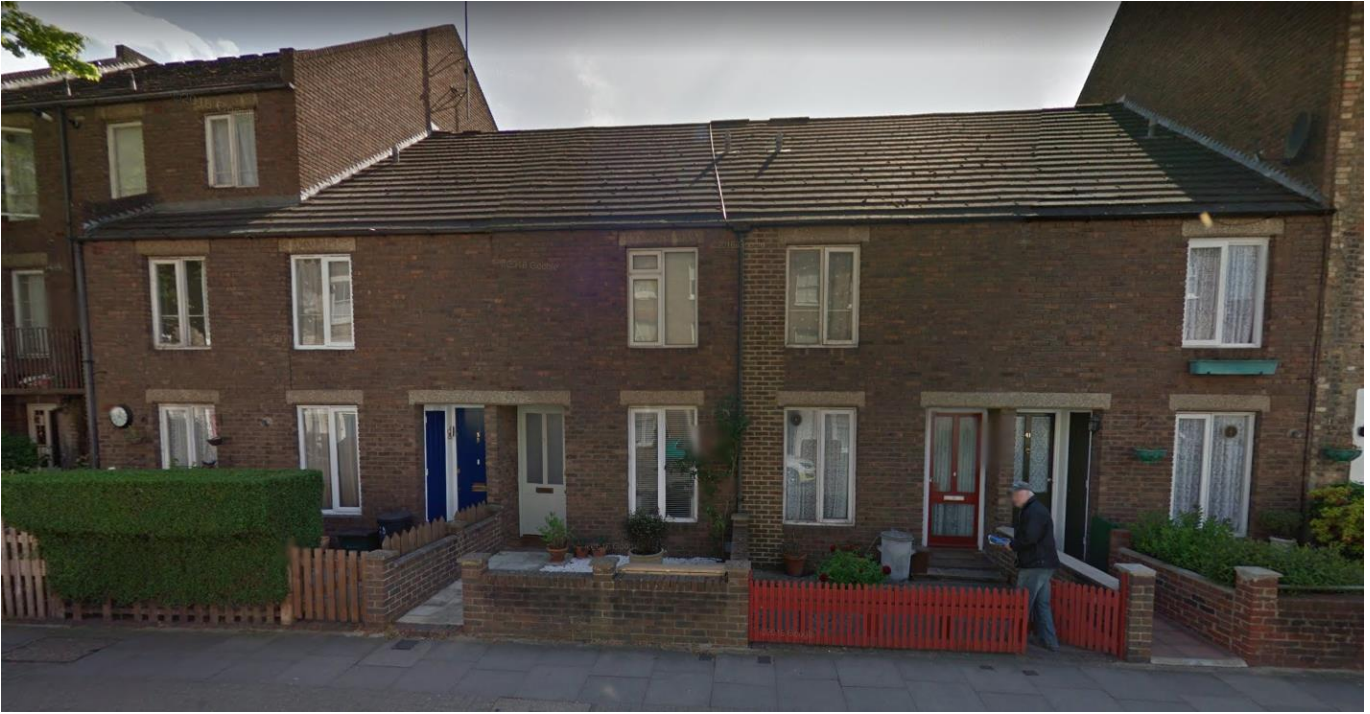
Image 5: Photograph of Nos 35-41 Charteris Road whose windows comprise a mix of timber and uPVC
