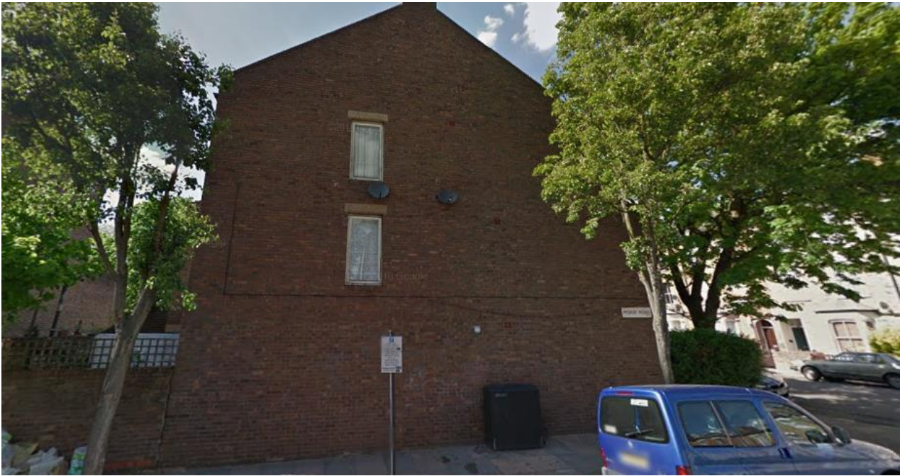
Image 3: Photograph of the side of the Site facing Moray Road
