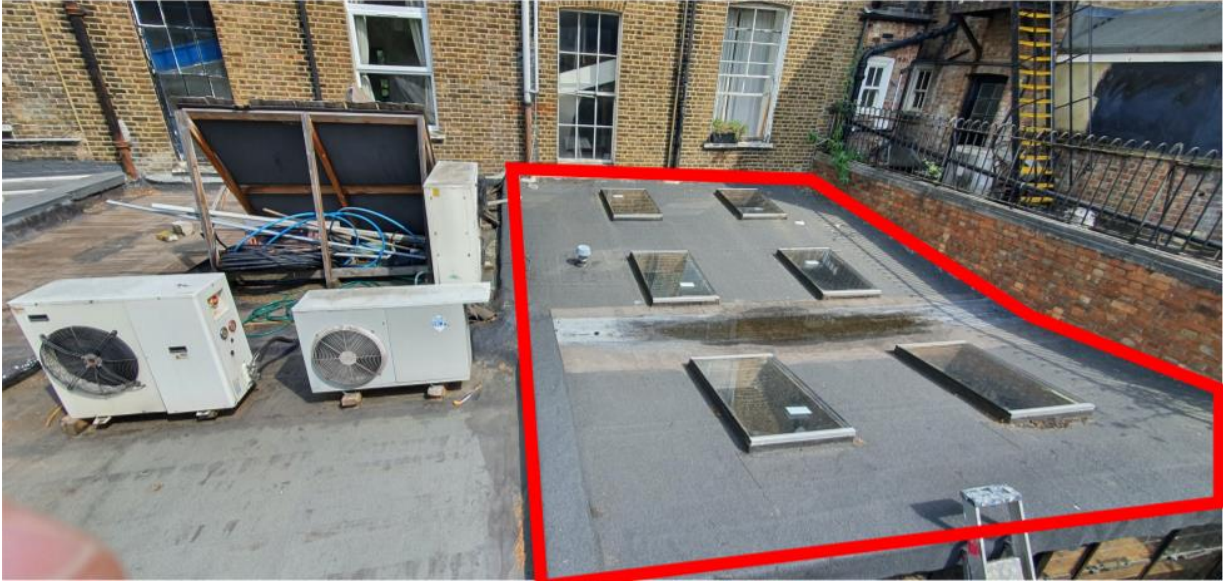
Image 3: View of roof of rear existing extension
