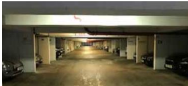
Image 4: Internal view of existing car park.
