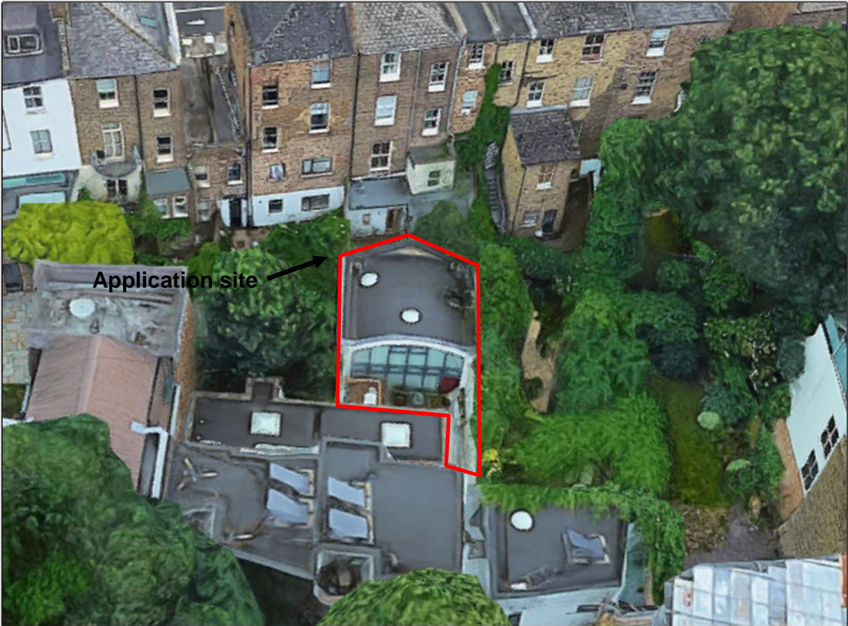
Image 1: Aerial view of the application site
