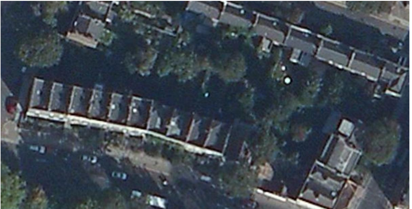
Image 1 - Aerial view of the site and surroundings
