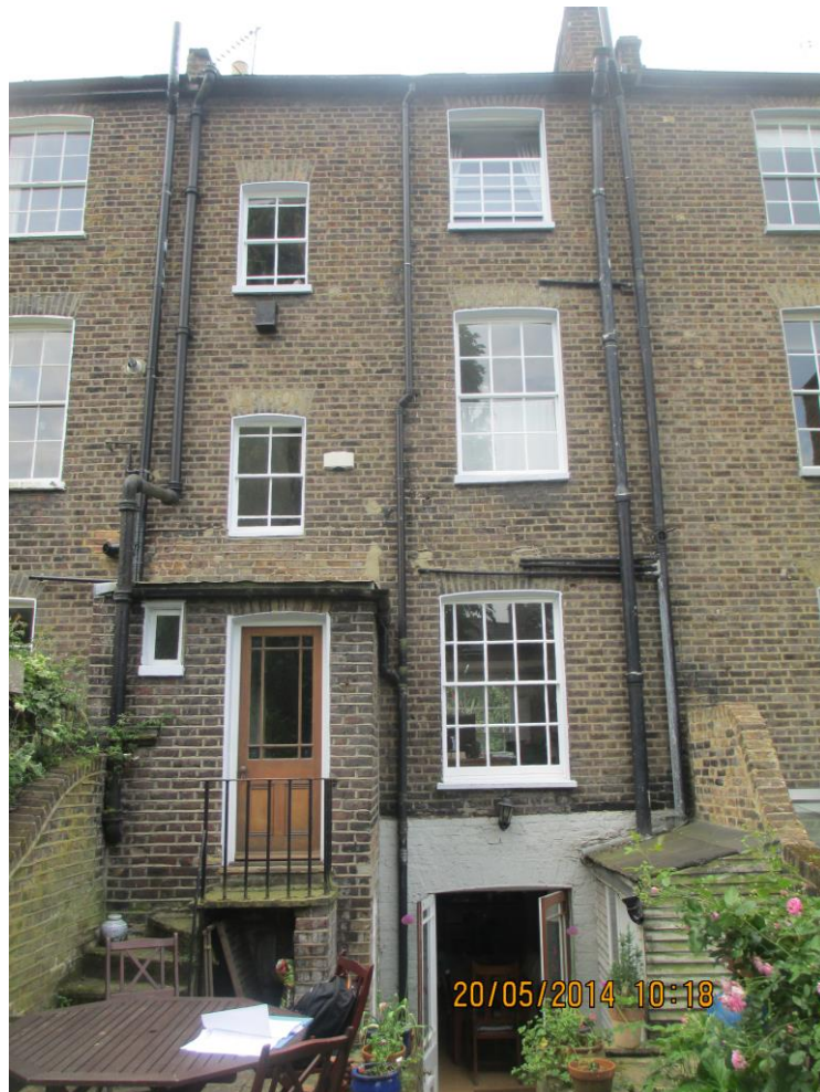
Image 2 - View of rear elevation of the site
