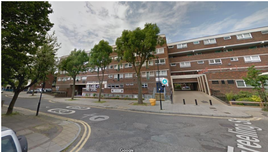
Image 2: Photo showing existing building
