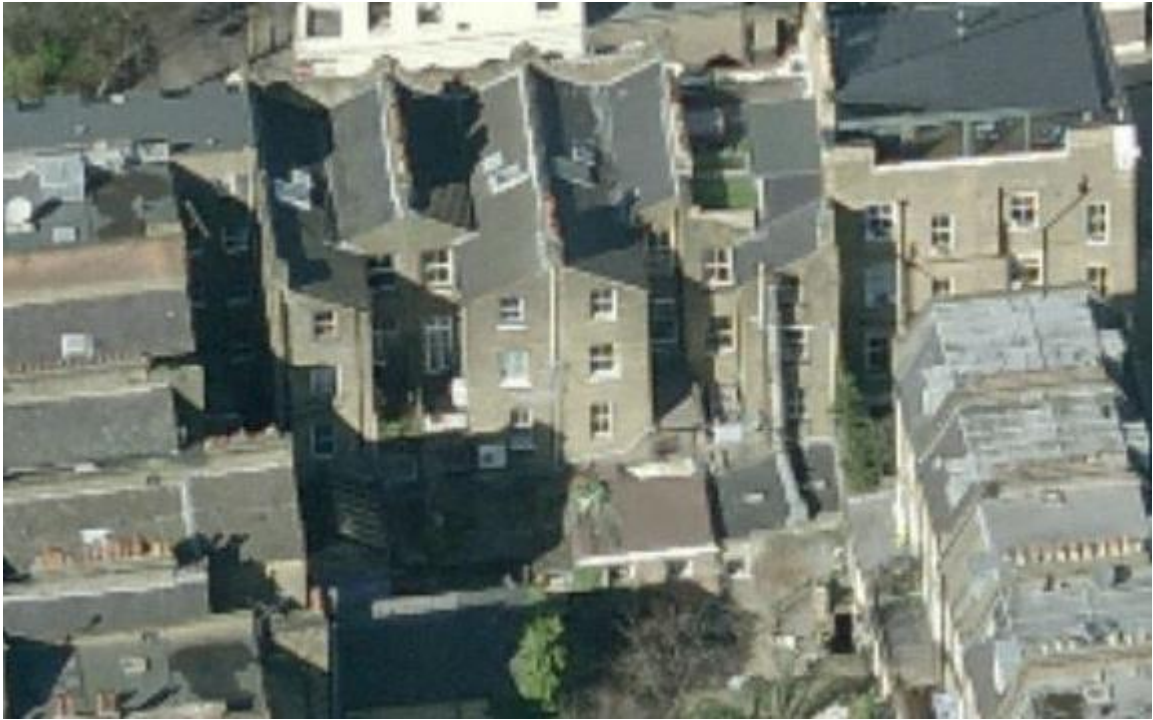
Image 1: Aerial view of the site and terrace setting.
