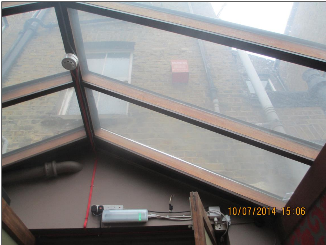
Image 3: Views of the 1 st floor rear elevation from within the rear section of the existing pub.
