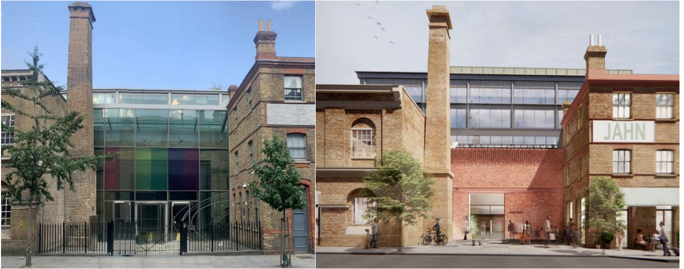
Image 1 – Existing and proposed elevations - Entrance to Jahn Court adjoining 34b York Way
