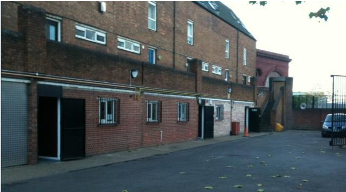
Photo 1: View of office space (previous undercroft)
