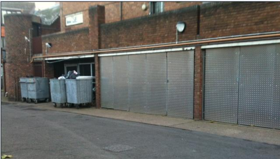
Photo 2: View of storage space (previous undercroft)
